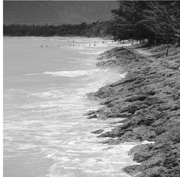
**Waimanalo, Oahu.** Sand impoundment behind this revetment at Bellows Airfield creates a local sand deficiency. As a result, it is responsible for ~1000 ft of beach loss and dune destruction, and chronic erosion characterizes the coast to either side of this structure.
