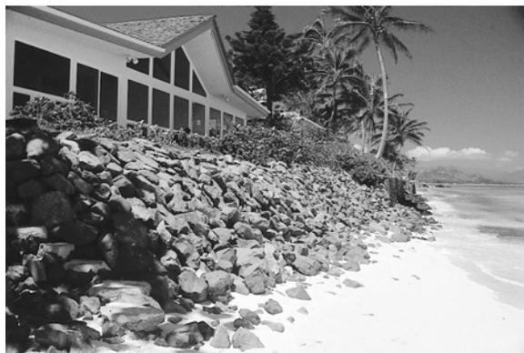
**Windward Oahu.** Coastal development, besieged by chronic erosion, has historically relied on shoreline hardening for protection. In many cases this has caused beach narrowing, beach and dune loss, and has restricted public access along miles of the Hawaiian coast. COEMAP provides a framework for decision-making and implementation to better manage the problem of coastal erosion and to improve the conservation of our beaches and dunes.
