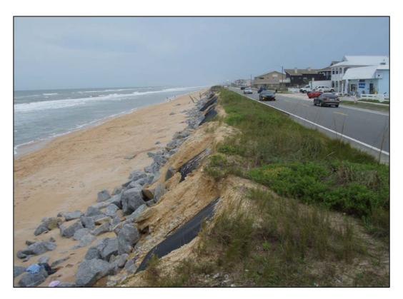
Figure G-4. Atlantic Ocean, beach, and reveted dune system fronting State Road A1A in the project area.
