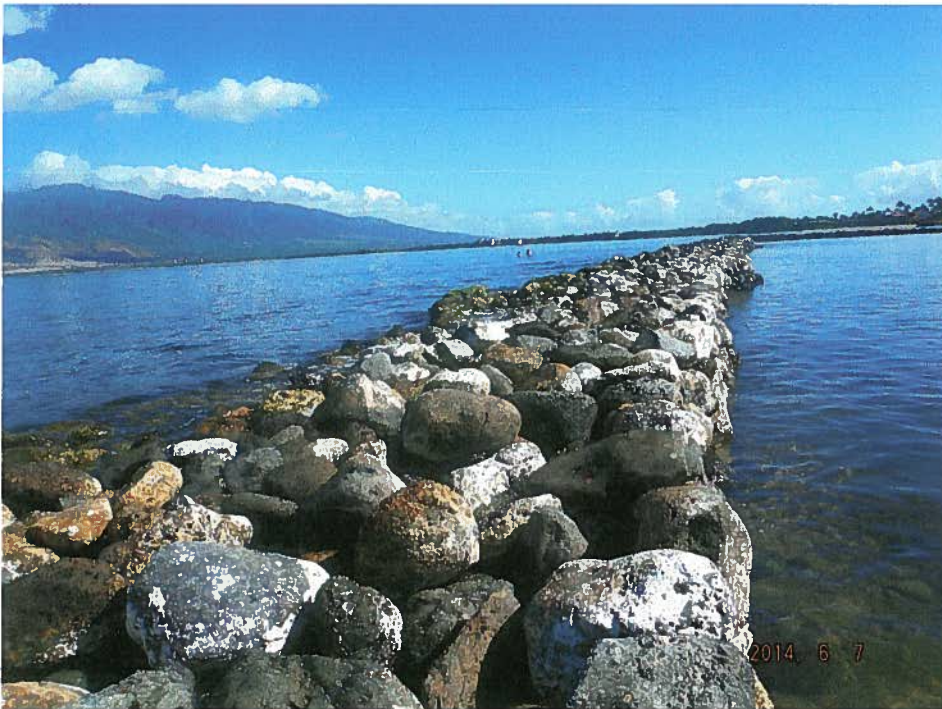
Figure 2. June 7, 2014 Western section of wall restored.
