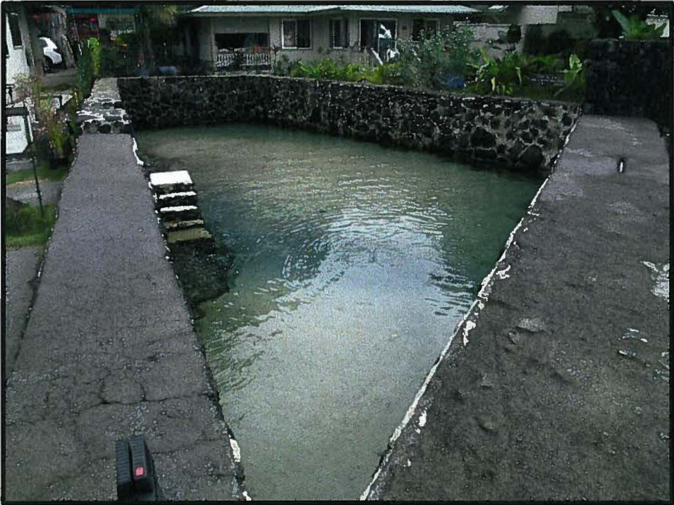
Photo 1. A photo of Kī'ope Fishpond at high tide, view to the southeast. Note, the large amount of sand accumulated at the bottom of the Fishpond, where at high tide the pond is less than 12 inches deep.
