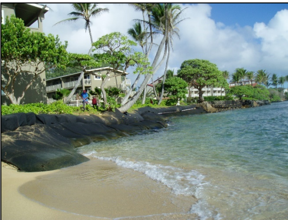
c) Photograph of Kauai Kailani beach following groin removal with emergency erosion protection taken on October 31, 2018
