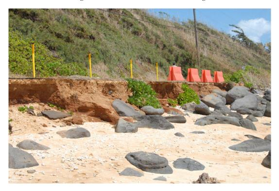
Figure 1-4. Undermining of the road
