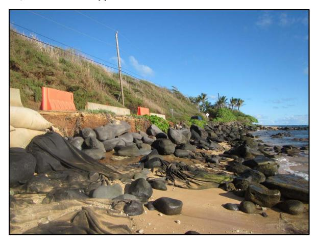
Figure 2. Photograph of the shoreline erosion undermining 'Aliomanu Road.
