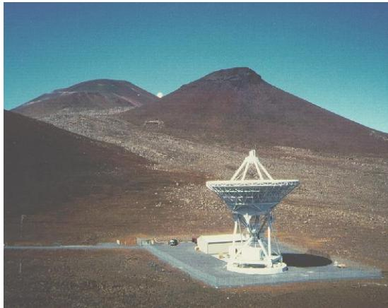
The Mauna Kea Very Long Baseline Array (VLBA) is one unit in an integrated system of ten identical radio telescopes stretching from the U.S. Virgin Islands to Hawai'i, which are operated remotely from Socorro, New Mexico. Each VLBA station consists of a 25m antenna and an adjacent control building. The ten stations work together as one single instrument. It is in the lower summit region at approximately 3700 meters elevation.
