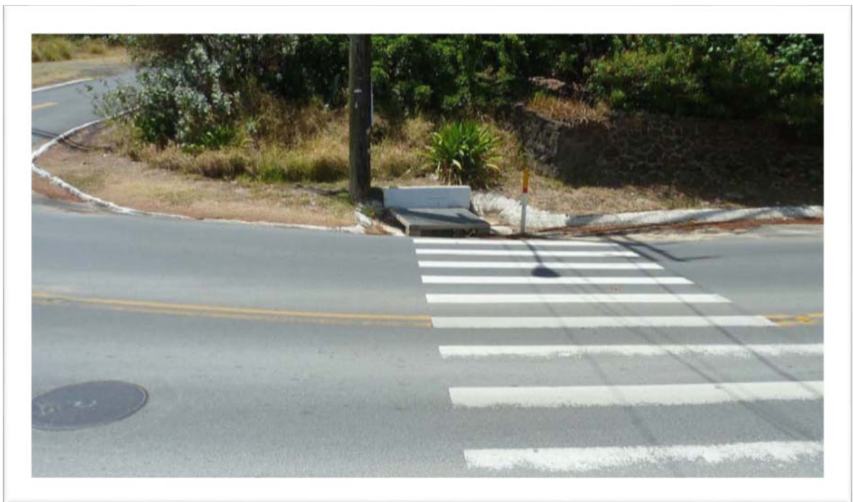
Figure 1-4. Road Drain Inlet near Alala Road – Kaneapu Place intersection
