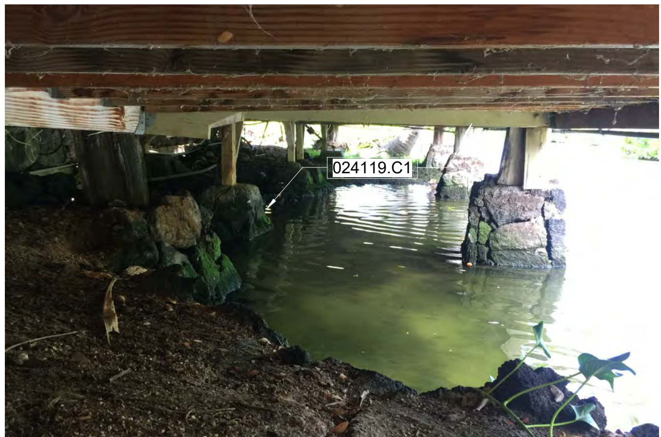
VIEW 1 - FOOTING UNDER STAGE
