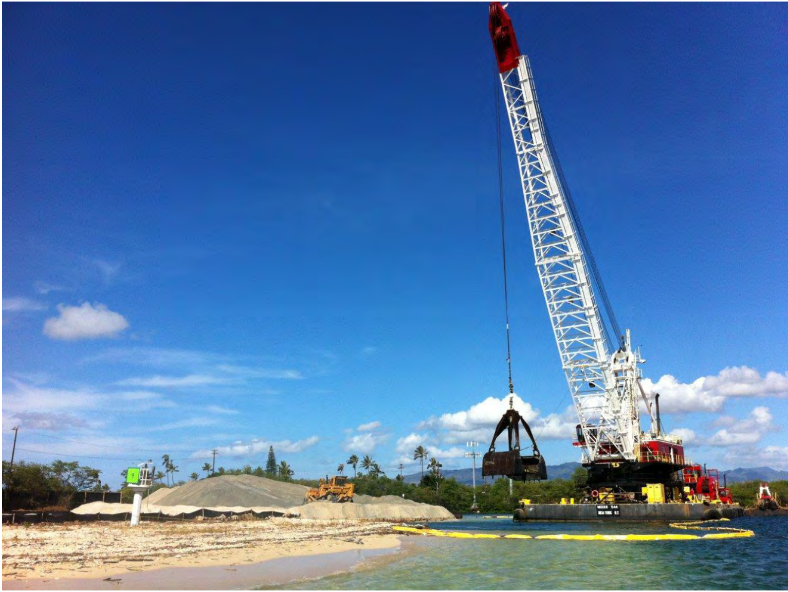
Figure 1-13. Clamshell bucket sand recovery at Pearl Harbor entrance channel.
