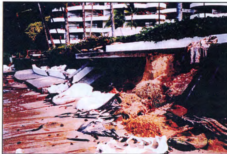
Figure 5-5 Beach loss and collapsed sidewalk at Sheraton Maui (March 24, 1998)
