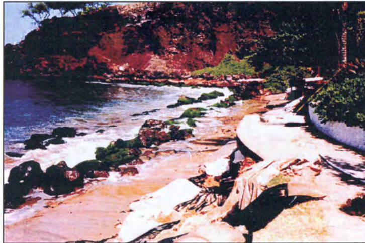
Figure 5-4 Beach loss and collapsed sidewalk at Sheraton Maui (March 24, 1998)
