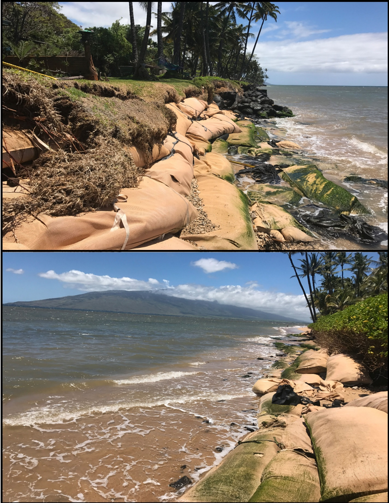
Figure 11. Halama Street Beach Loss (Top: Updrift, Bottom: Downdrift)
