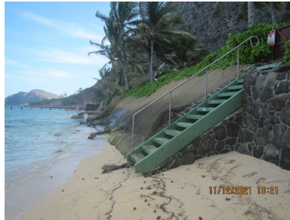
Photograph #14 (Nov 2021): Photograph of stairs and temporary emergency erosion control structure seaward of TMK (1) 4-1-001:009
