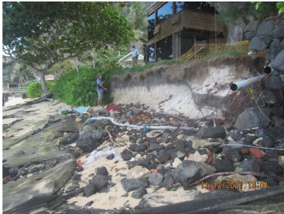
Photograph #13 (Nov 2021): Photograph of deflated temporary emergency erosion control structure and collected debris fronting TMK (1) 4-1-001:012
