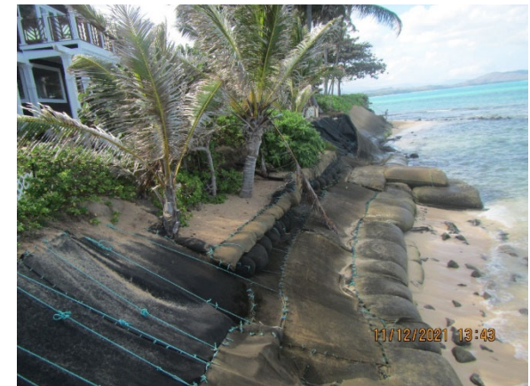
Photograph #12 (Nov 2021): Photograph of temporary emergency erosion control structure fronting TMK (1) 4-1-001:008
