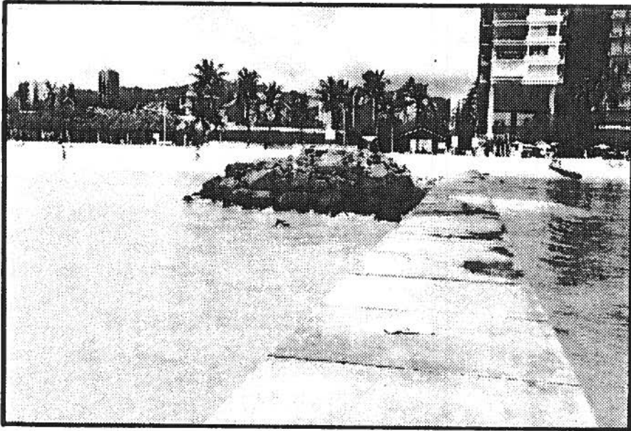
PLATE 7 KALIA RELIEF DRAIN LOOKING MAUKA
