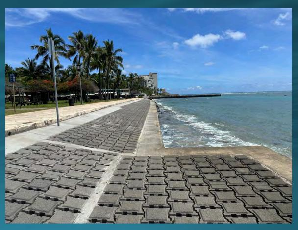
There is a 98-foot long protrusion along this section of the seawall that extends between twelve and twenty-seven feet seaward. Some records refer to it as a "planter box," while oral accounts state that it is a remnant of the public baths. The area was capped with concrete pavings in 2020. Waves frequently overtop the wall during the summer south-swell season. The Publics surf break is offshore.
