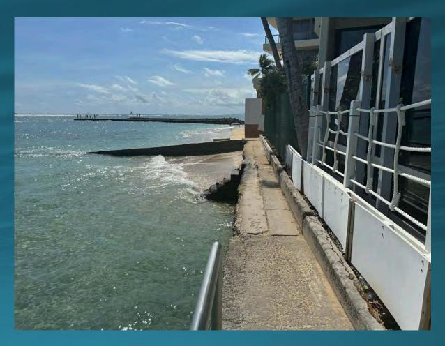
The walkway fronting the Halekūlani and Outrigger hotels is in a state of disrepair, although it is still frequently used by pedestrians. There are no alternate routes through the hotel properties to reach Fort DeRussy. The first seawalls in Waikīkī were built here in the 1890s and 1900s in response to changing currents and increased erosion, perhaps due to the dredging of the Halekūlani Channel. There are remnants of eight small groins that were once placed here to stabilize the beach.
