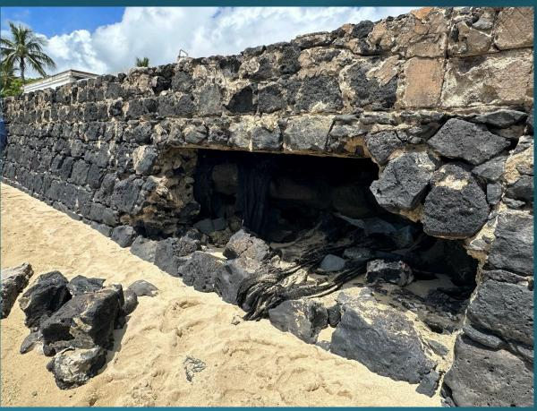
There is a shallow reef flat offshore extending approximately 35 yards, then a channel that was dredged in the 1930s to create a swimming basin. A narrow beach has formed fronting the seawall. The beach appears some years, and disappears other years. Parts of the seawall are failing, and the walkway is currently closed.
