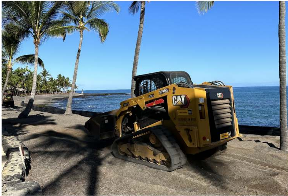
Figure 2-1 Skid steer used to transport sand to placement area
