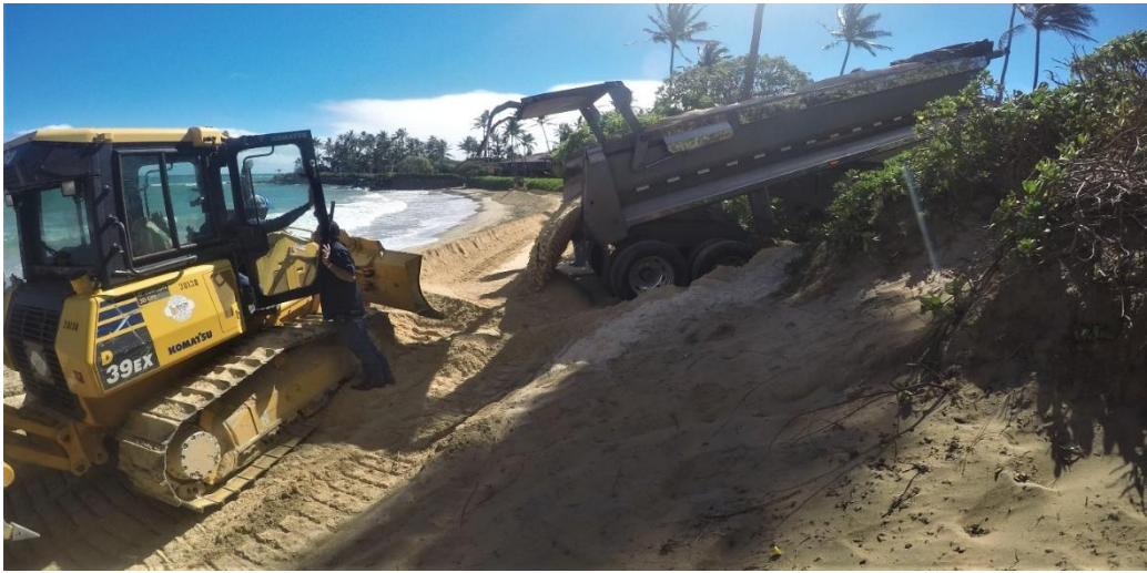
Figure 7-1. Dump truck delivering sand to the west end of the cove for placement on the berm (Maintenance #4)
