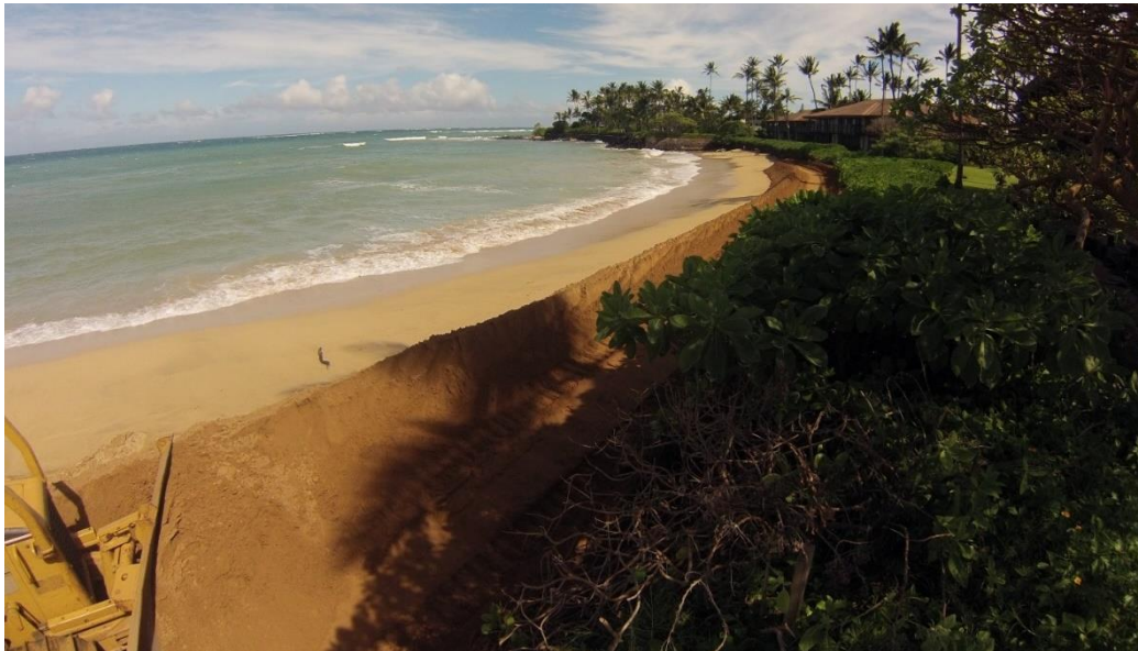
Figure 4-4. Sand grading on the berm (Maintenance #1)
