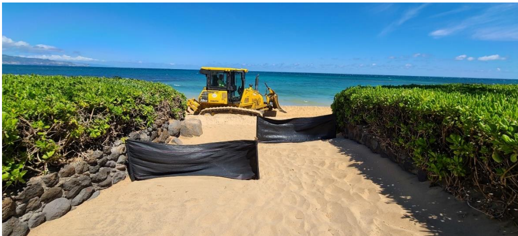
Figure 6-2. Bulldozer spreading sand along the berm (Maintenance #3)
