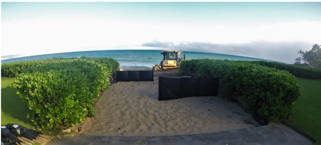
Figure 7-2. Bulldozer spreading sand along the berm (Maintenance #4)
