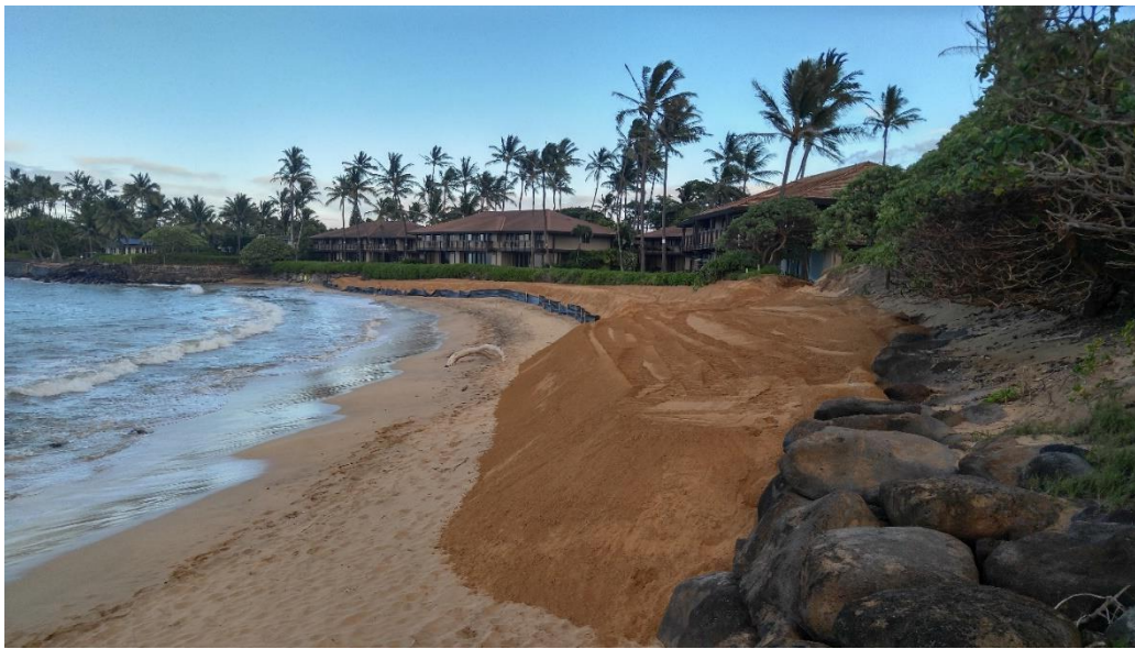
Figure 5-5. Beach and berm condition after placement on September 7, 2016 (Maintenance #2)
