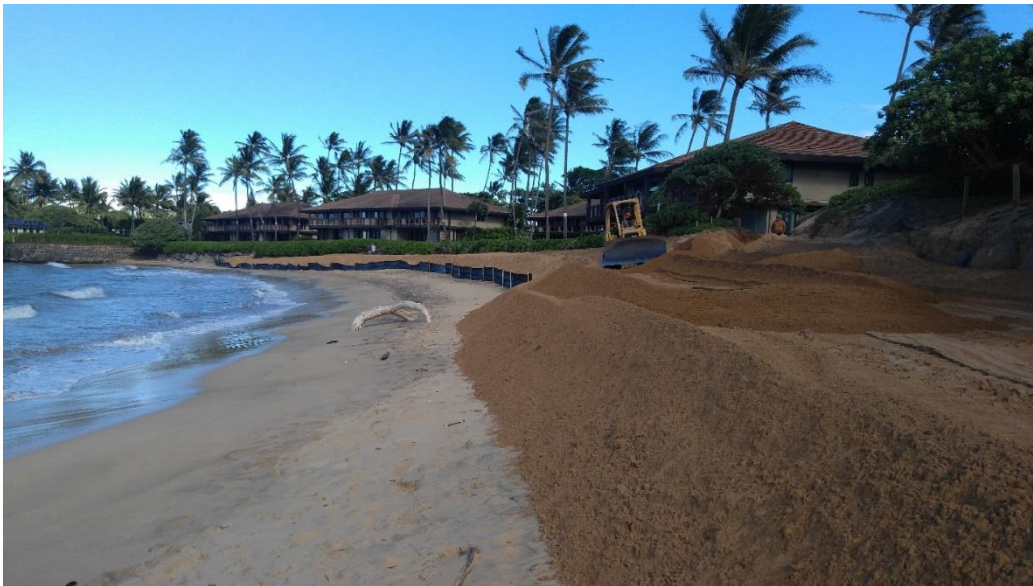
Figure 5-2. Bulldozer spreading sand along the berm (Maintenance #2)
