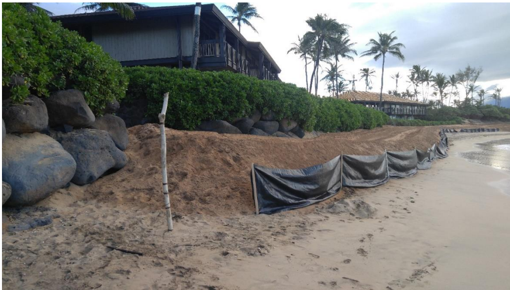
Figure 5-3. Graded sand with finished makai slope and silt fencing ending near Transect 3 (Maintenance #2)
