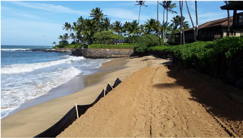
Figure 4-5. Graded sand with finished makai slope and silt fencing ending near Transect 3 (Maintenance #1)
