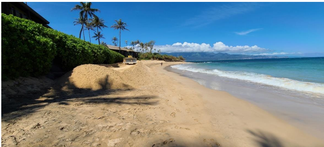
Figure 6-3. Graded sand with finished makai slope and silt fencing ending near Transect 3 (Maintenance #3)
