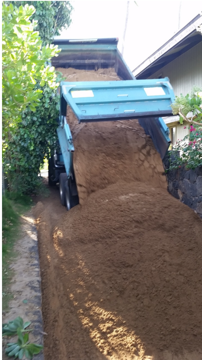
Figure 4-2 Smaller dump truck delivering sand to the County of Maui beach access path
