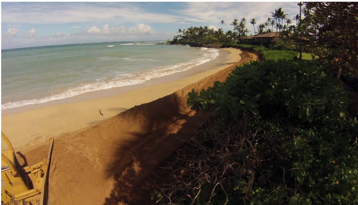
Figure 4-4 Sand grading on the berm
