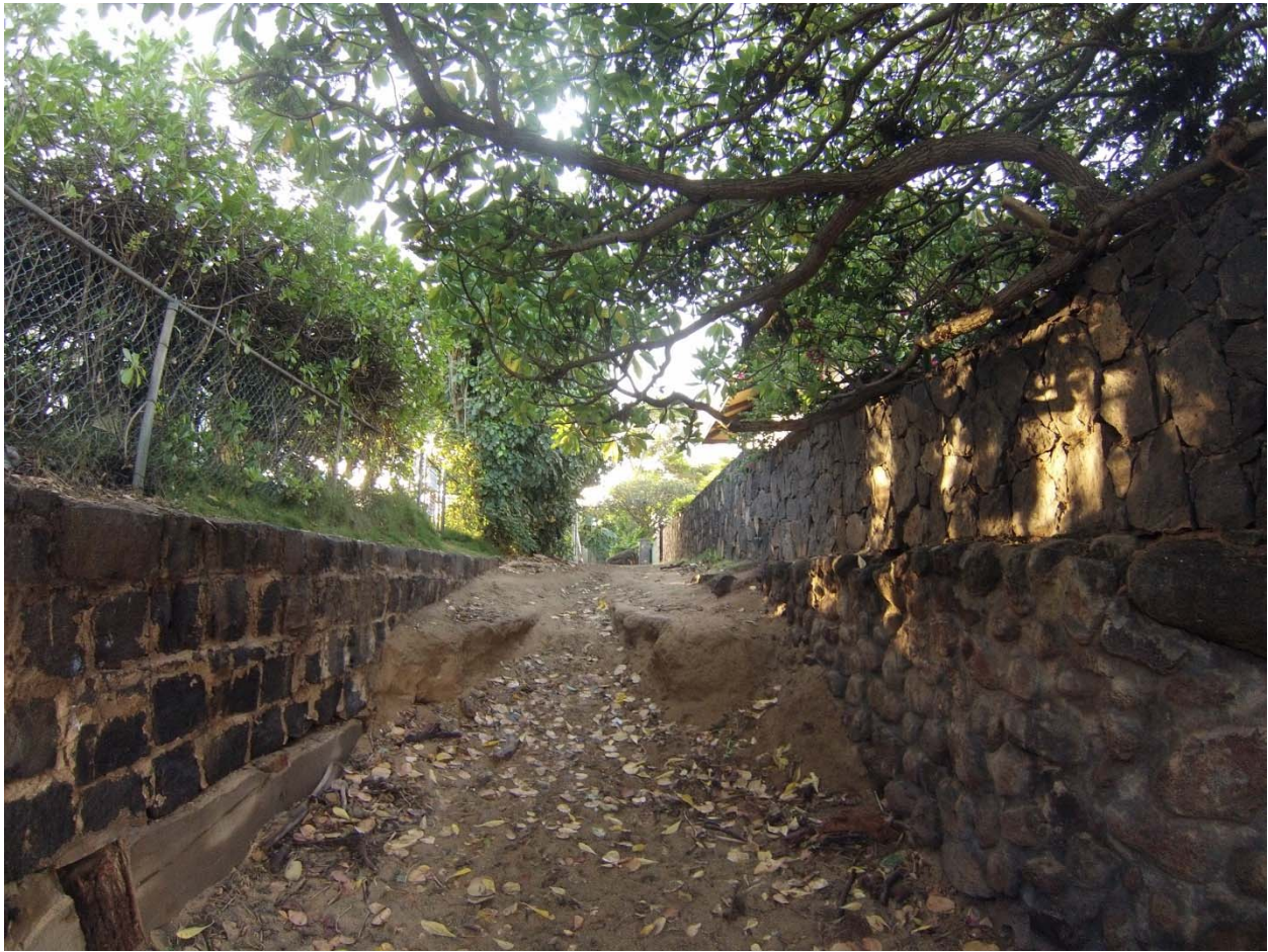
Figure 4-9 Three foot scarp in County of Maui beach access path
