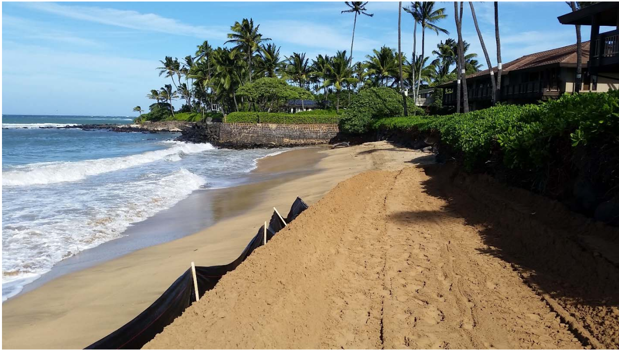
Figure 4-5 Graded sand with finished makai slope and silt fencing ending near Transect 3
