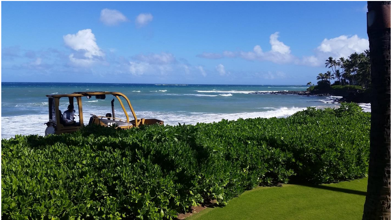
Figure 4-3 Bulldozer spreading sand along the berm (Maintenance #1).
