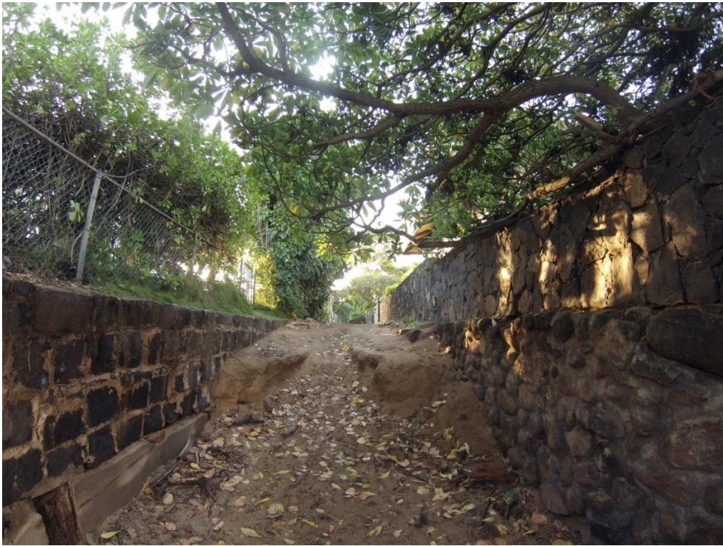
Figure 4-9 Three-foot scarp in County of Maui beach access path (Maintenance #1).
