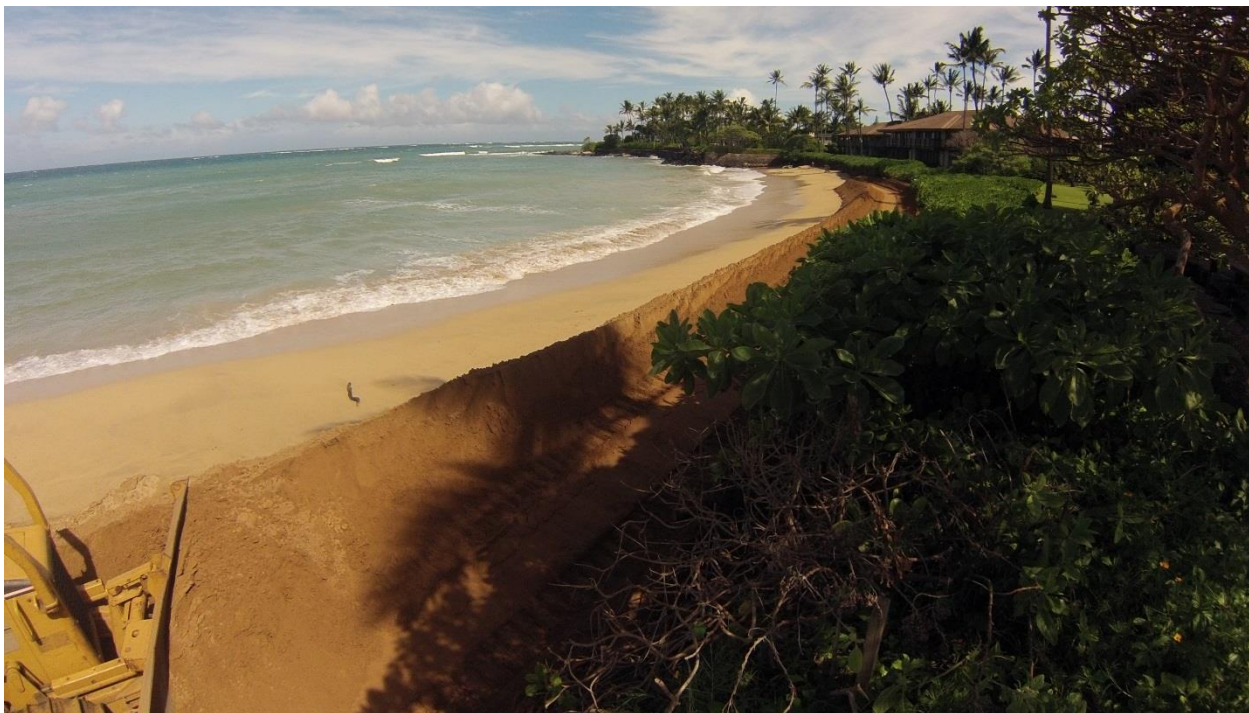
Figure 4-4 Sand grading on the berm (Maintenance #1).
