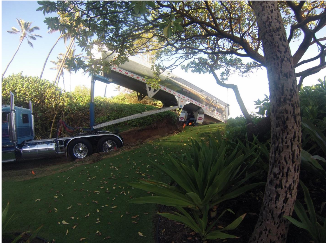
Figure 4-1 Dump truck delivering sand to the west end of the cove for placement on the berm (Maintenance #1).
