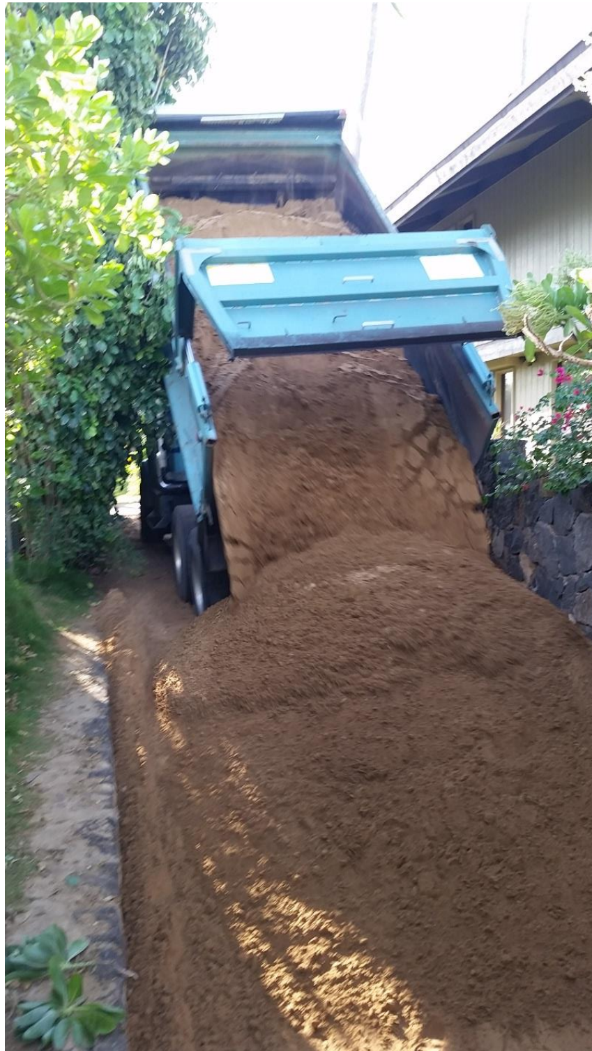
Figure 4-2 Smaller dump truck delivering sand to the County of Maui beach access path (Maintenance #1).
