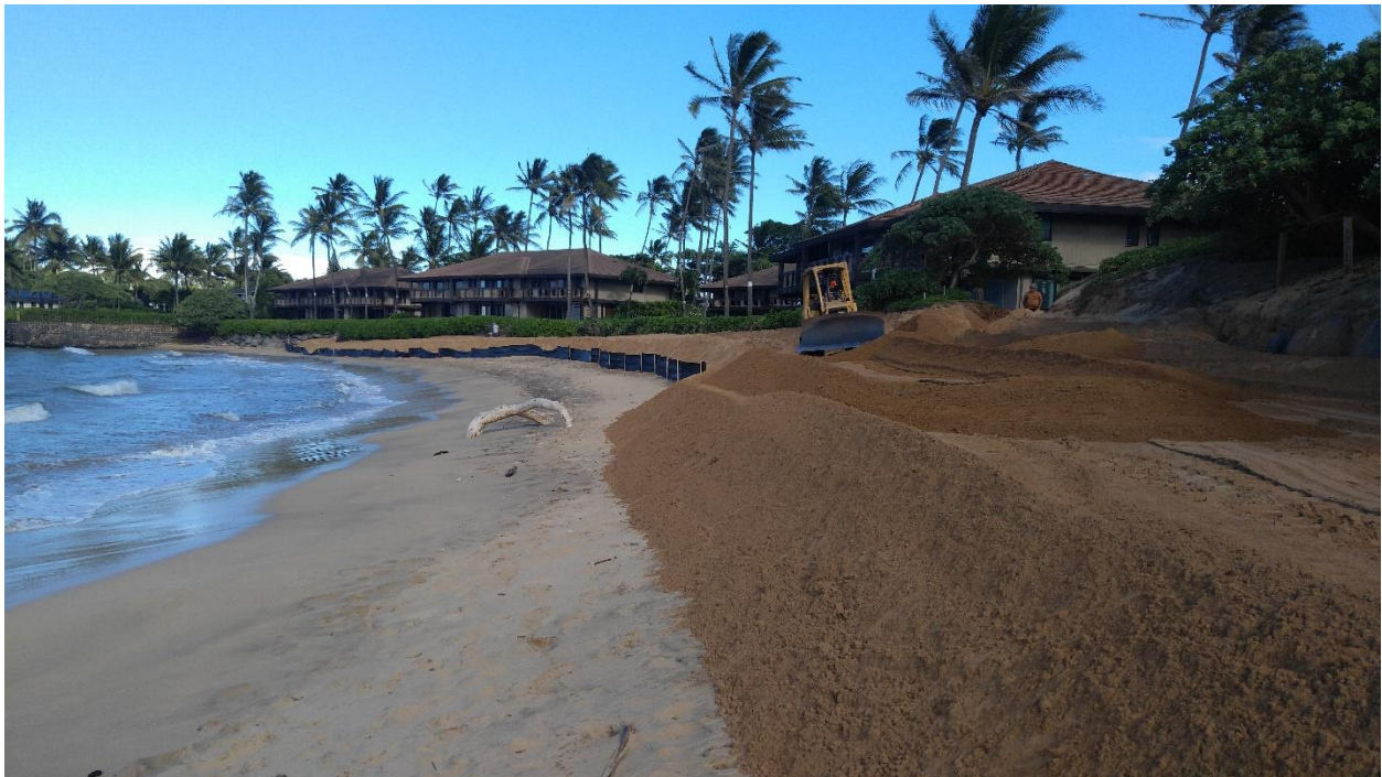
Figure 5-2 Bulldozer spreading sand along the berm (Maintenance #2).
