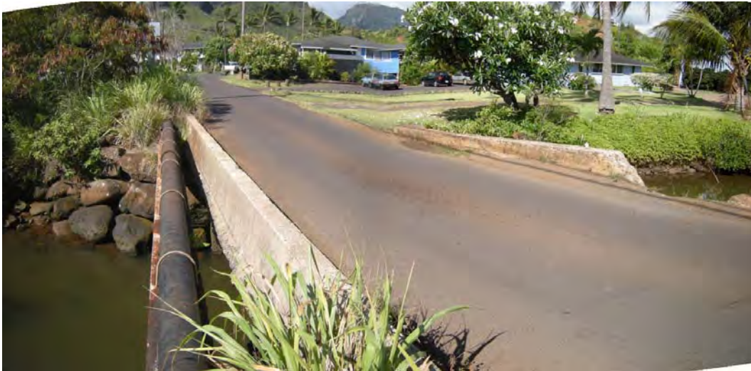
Figure 9. Niumalu Bridge, view facing south. Note the original curb on the right (west curb) and the replacement curb on the left (east curb).
