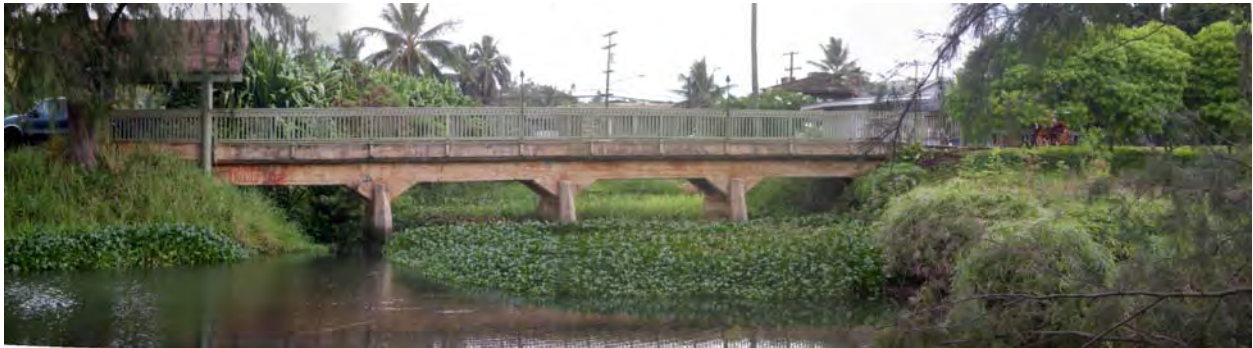
Figure 3. Nawiliwili Stream Railroad Bridge, view facing west. Note the three battered piers supporting haunched girders, added wood balustrade, and added roof cover at left (south) end.
