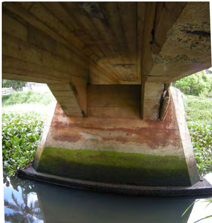
Figure 4. Underside of Nawiliwili Stream Railroad Bridge, underside view facing north. Note the pier with battered tapering faces, haunched girders, and board formed surface.
