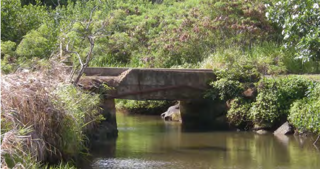
Figure 8. Niumalu Bridge view facing east, showing the original (west) curb with broken section and mis-aligned iron pipe.
