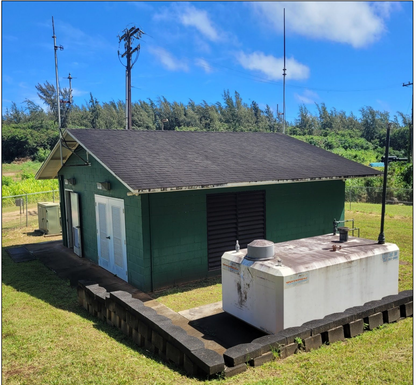
Figure 10: Example of a Similar Pump Control and Chlorination Building
