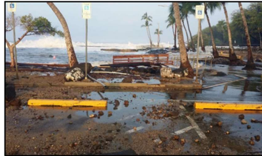
(d) January 2015. Parking lot during storm conditions. Waves can be seen overtopping main breakwater, resulting in flooding of parking lot.
