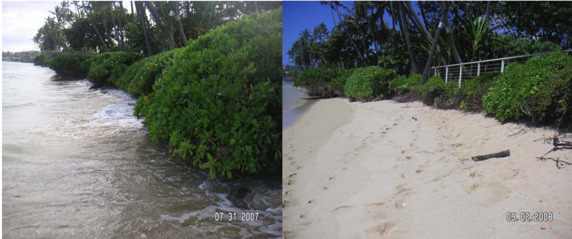
FIGURE 21. Encroaching dune vegetation can create an overhang and unsafe conditions during erosion events and severely restrict lateral public access. Images show before (left) and after (right) encroaching vegetation was managed and trimmed back to reopen the beach. (Photos: Lucinda Pyles)
