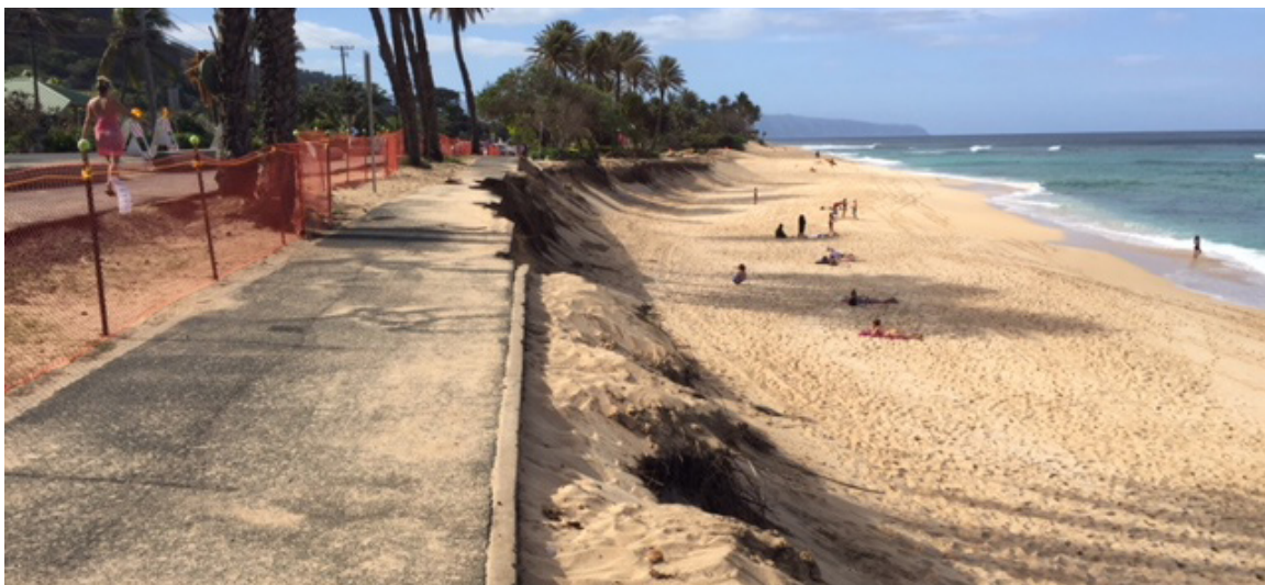
FIGURE 14. Sunset Beach, along O’ahu’s North Shore, demonstrates substantial erosion of the dune and the destruction of a walkway following a strong swell event in 2018.
