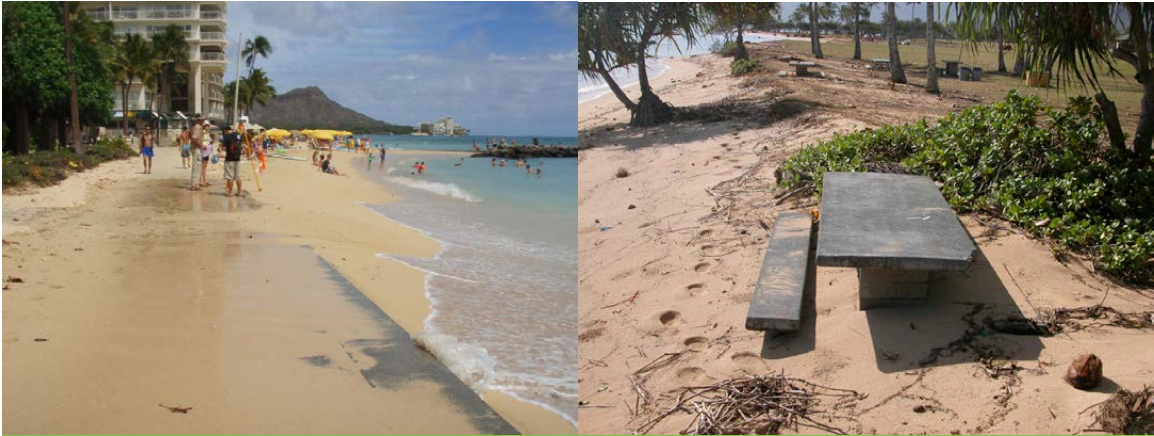
FIGURE 29. Sand can be a maintenance problem for areas where walkways (left, Waikiki Beach) or other infrastructure (right, Kualoa Park) get covered by wind- or wave-driven sand migration.
