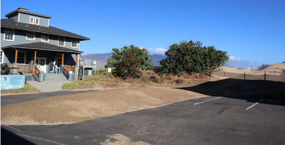
FIGURE 18. Sand blowing into parking areas or roadways presents a major management problem in Kihei, Maui.
