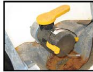
A 2" threaded ball valve is attached near the bottom of the tote
