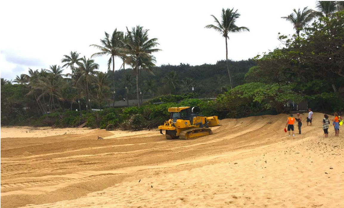
FIGURE 27. Sand pushing has been used at ‘Ehukai Beach, O‘ahu, and while not always necessary for a successful dune project, it is an option to quickly restore a dune.
