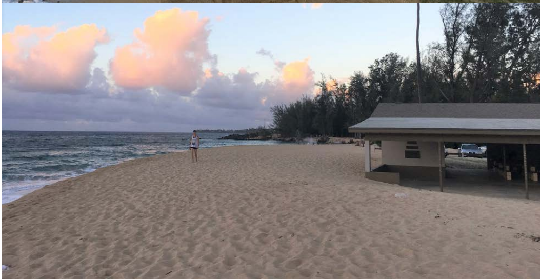
FIGURE 34. (Top) The Kapukaulua (Baldwin Beach) Pavilion is impacted by high waves during the peak seasonal beach erosion in the summer. (Bottom) The beach in front of the pavilion recovers as a result of winter season swells that push sand back toward the pavilion.
