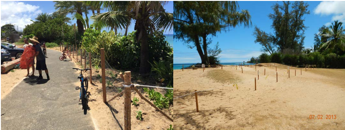
FIGURE 20. Fencing to delineate restoration areas and manage access can be as simple as wooden posts and rope, like these examples from Sunset Beach, O’ahu (left) and Lower Pā’ia Park on the north shore of Maui (right). In some cases, available wood sources can be repurposed for the job, as was done for the Sunset Beach fence project, which used invasive Ironwood trees that were cut down nearby.
