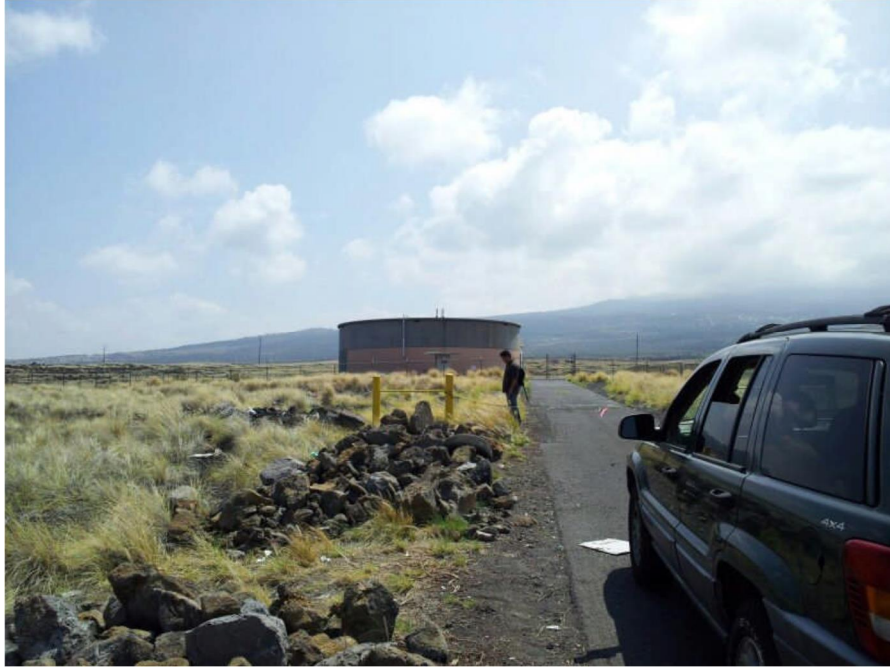
View of a water tank located east-northeast of the subject property.
