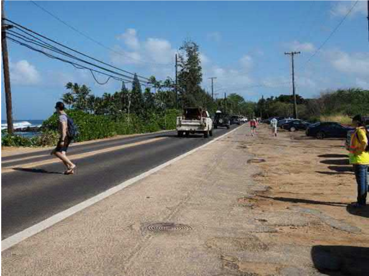
Figure 3-1. Kamehameha Highway – Existing Street View
