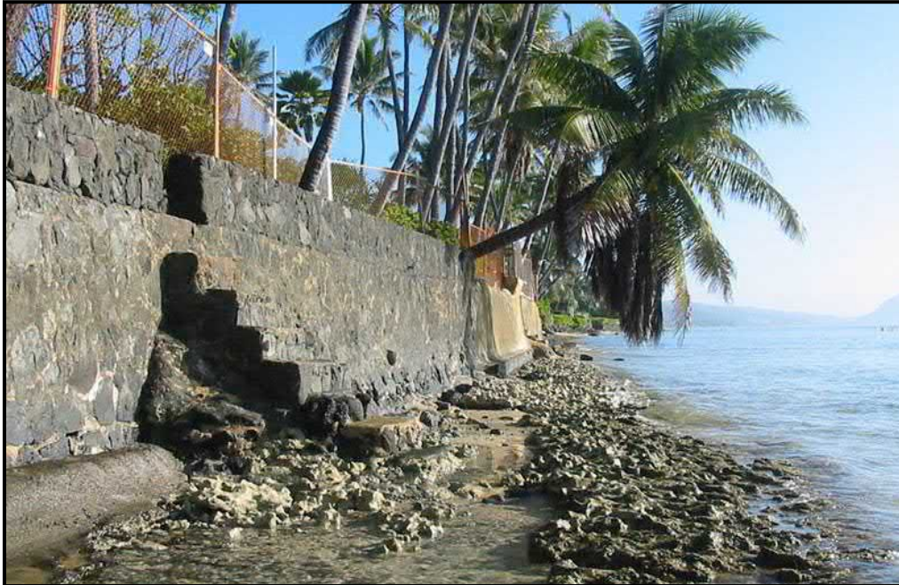
Figure 5-3. CRM seawall in Kahala
