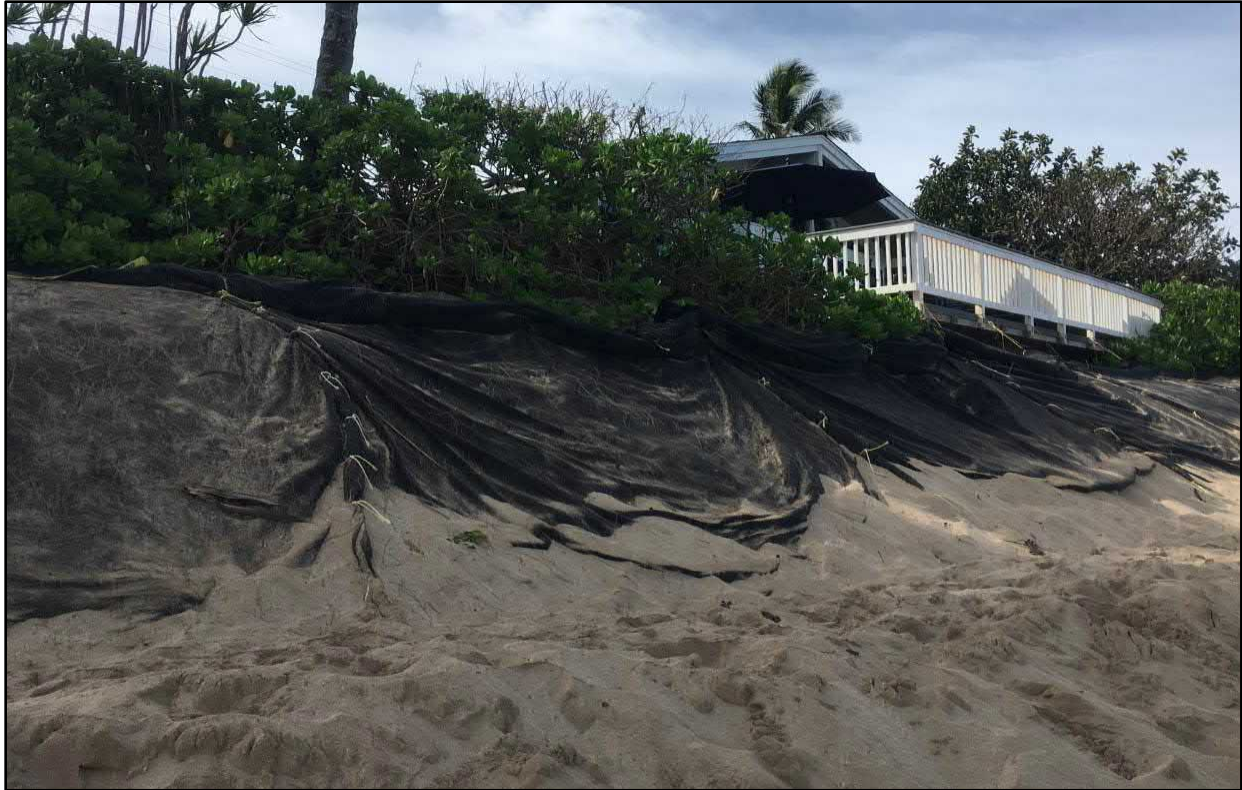
Figure 2-21. Geotextile drape protection for the storm berm
