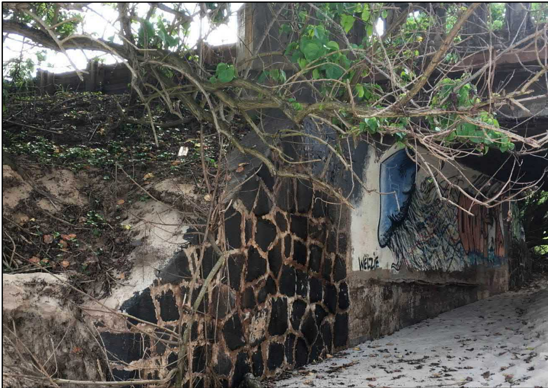
Figure 2-19. North bridge abutment
