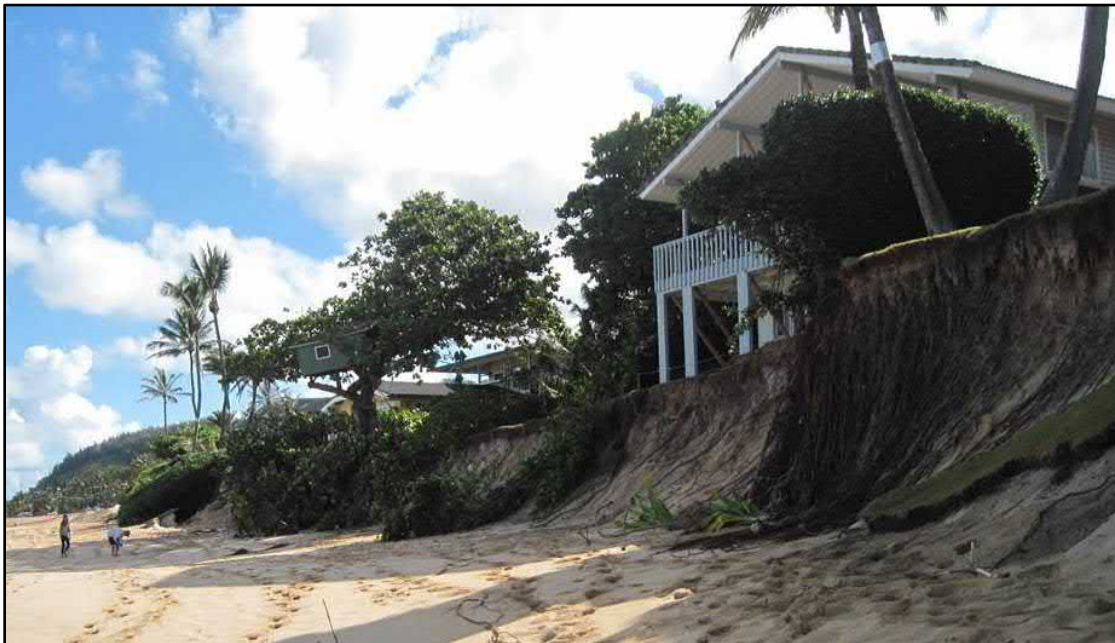
Figure 5-1. Storm berm collapse at Ke Nui Road, October 2013
