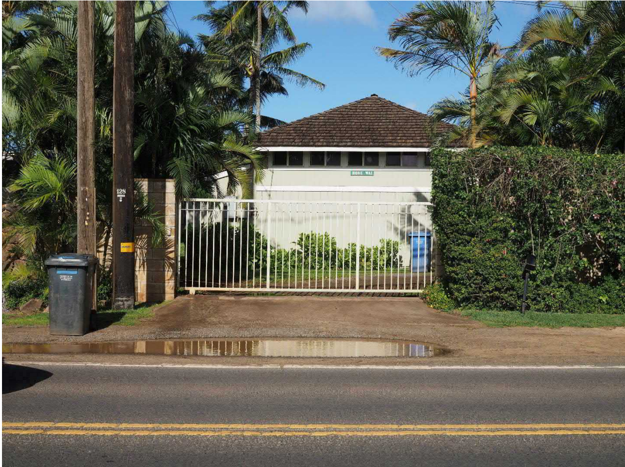
Figure 2-2. Typical Existing Makai Side View from Kamehameha Highway in the Project Area
