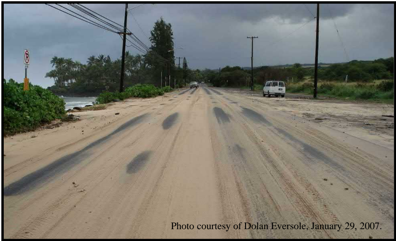
Figure 1-2. Photograph of Sand Deposition from Waves Overtopping Kamehameha Highway at Laniakea Beach
