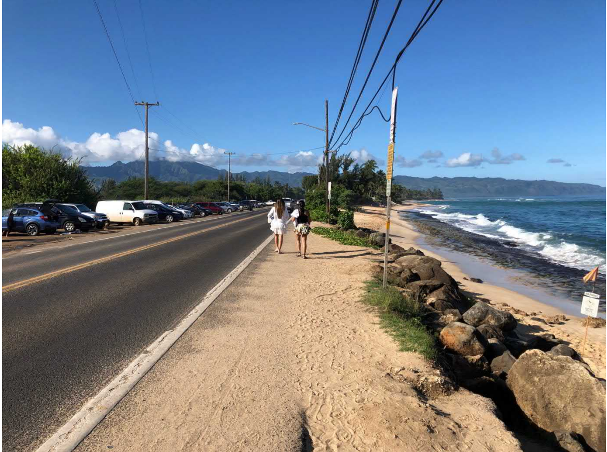
Figure 7. Existing highway is in close proximity to the coastline that is sparsely vegetated with pohuehue vines, invasive grasses, and trees such as milo, kiawe, and tree heliotrope.
