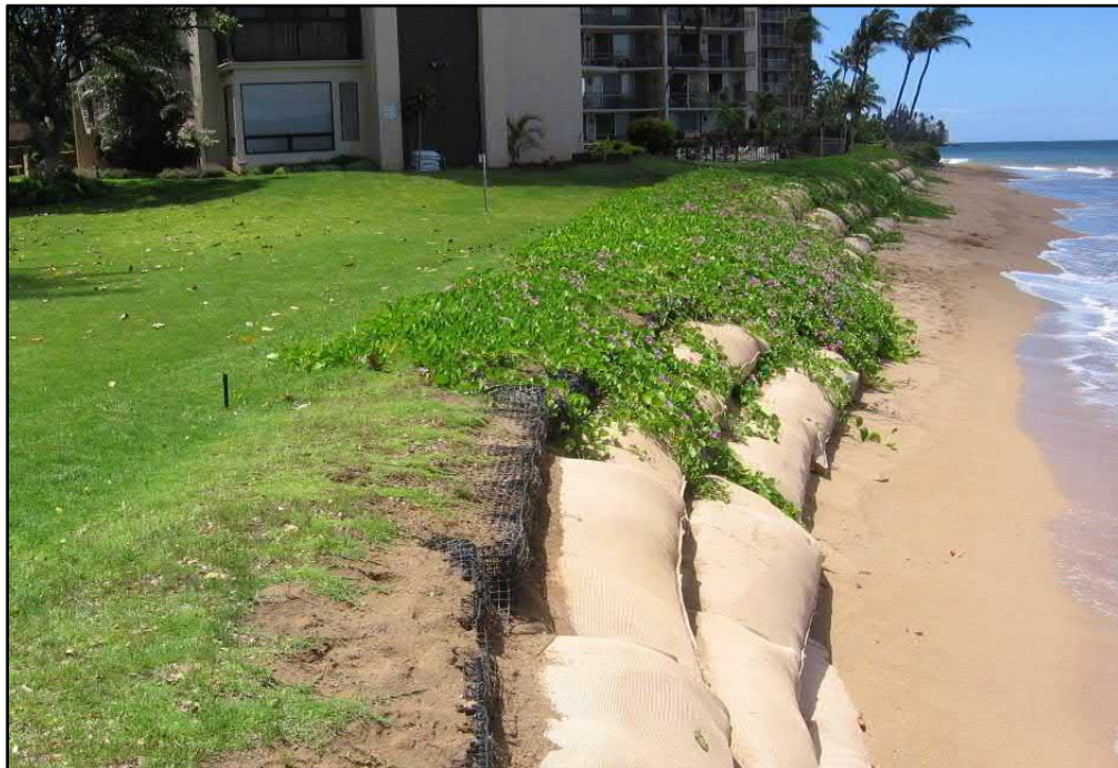
Figure 5-7. Rock-filled HDPE mattresses with fill and vegetation
