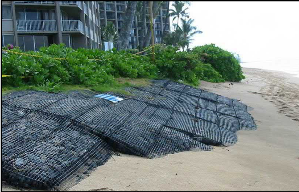
Figure 5-6. Rock-filled HDPE mattresses used for articulating protection
