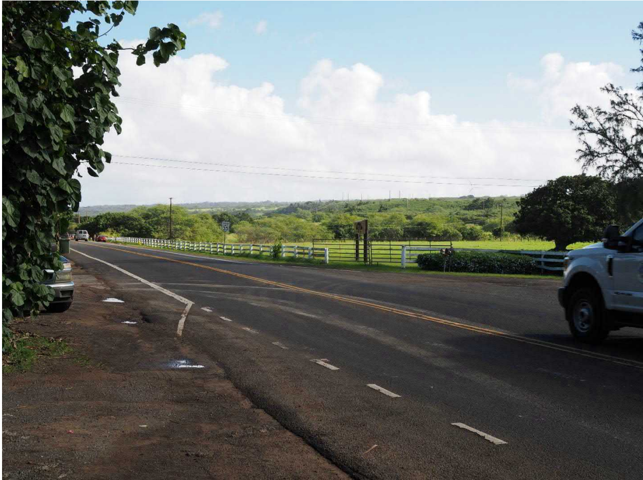
Figure 2-1. Typical Existing Mauka Side View from Kamehameha Highway in the Project Area
