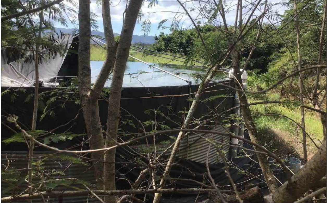
Photo 7. Overflowing Water Tank Upland about 1000 Feet above the Study Area that Contributed to Water Ponding at the Mouth of the Laniakea Stream Bed next to the Study Area
