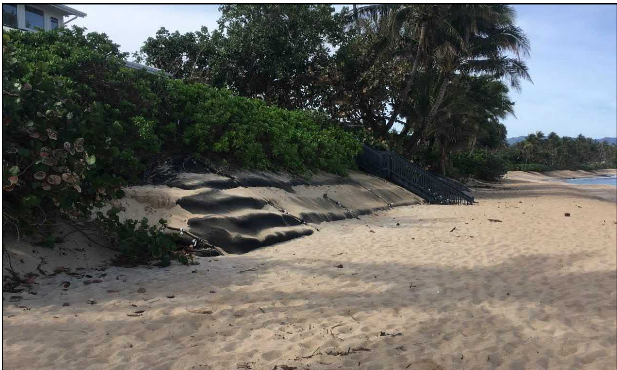
Figure 2-22. Geotextile drape storm berm protection
