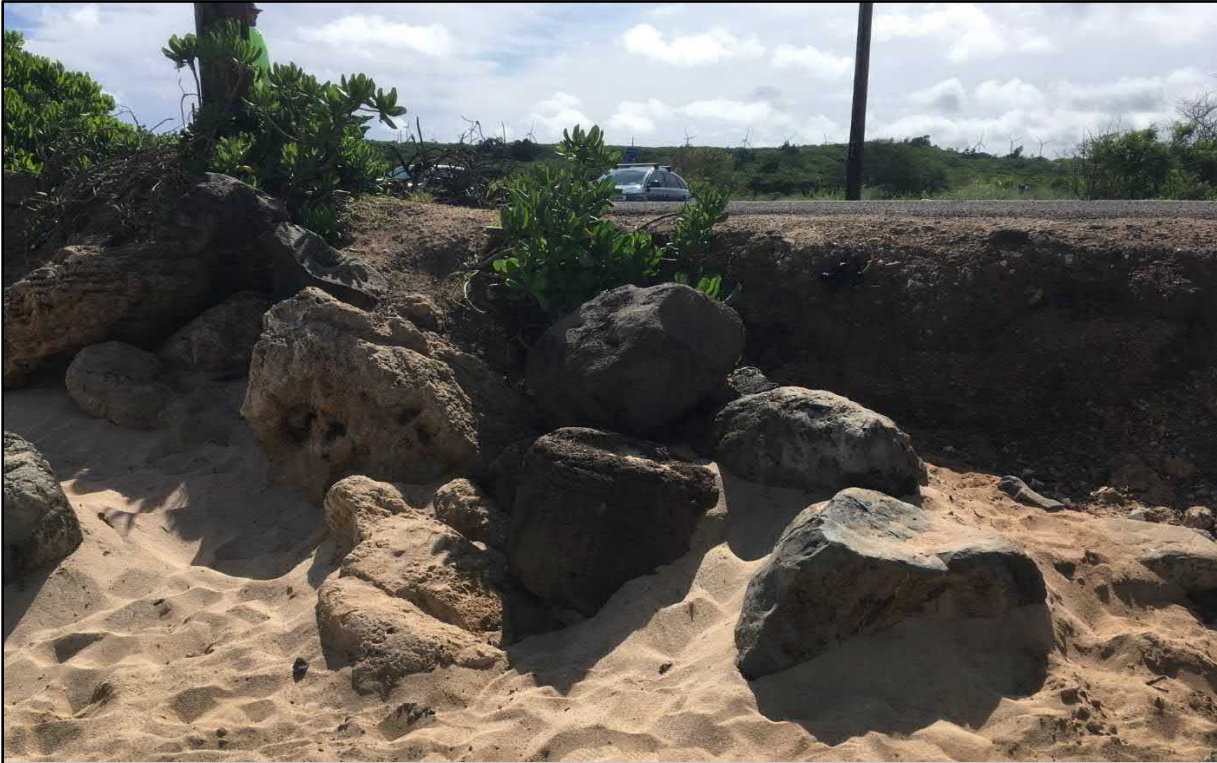
Figure 2-17. Scattered boulders mark the end of the rock revetment
