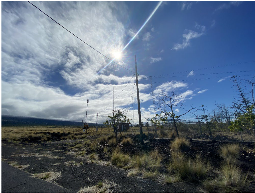
Looking SE at Proposed Site Location
