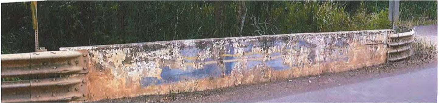
Photograph 6. HI_MauiCounty_HonoluaStreamBridge_0006. Parapet on the upstream side of the bridge. View facing southeast.
