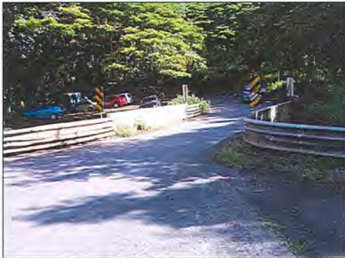
Figure 4. Honolua Stream Bridge view NNE from Highway 30.
