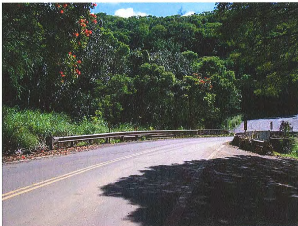
Photo 1 – Existing Honolua Bridge looking south
