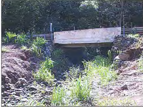
Figure 3. Honolua Stream Bridge view E from streambed.
