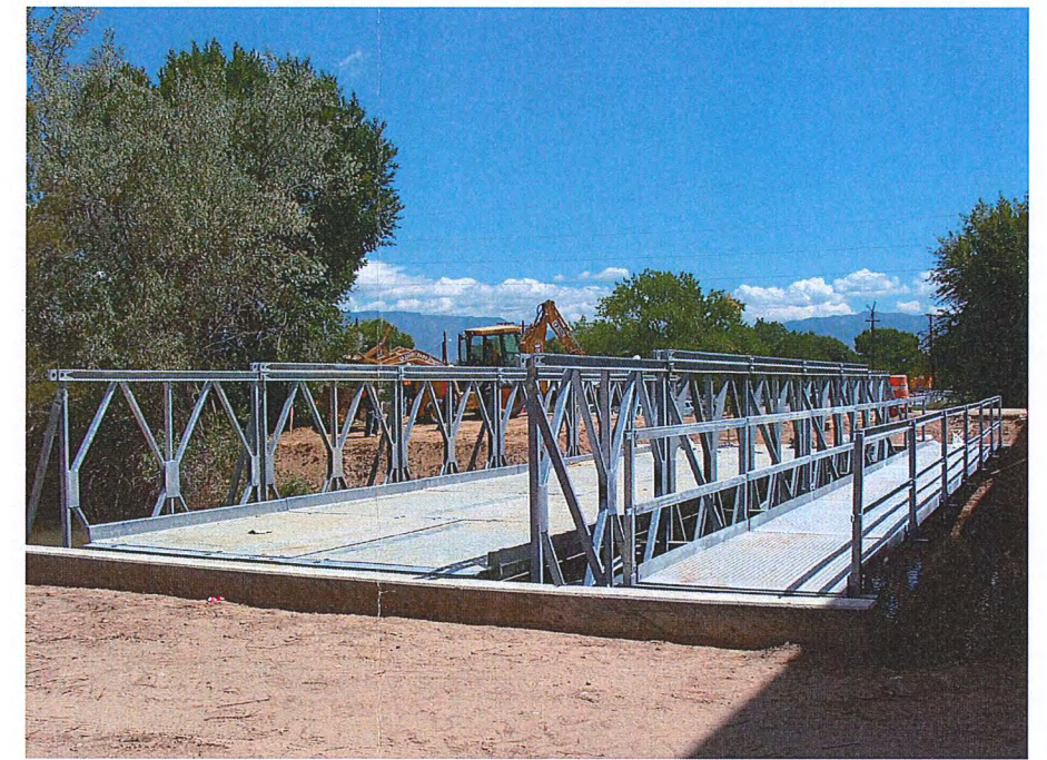
Temporary Bridge and Pedestrian Walkway
