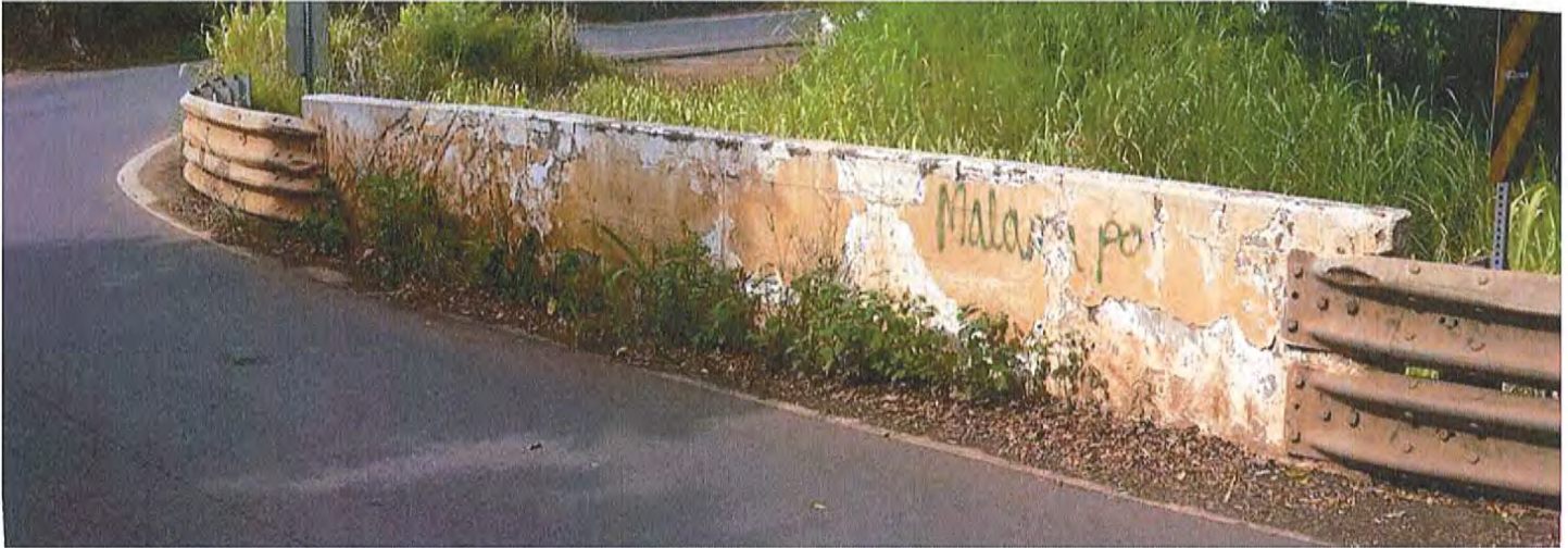
Photograph 5. HI_MauiCounty_HonoluaStreamBridge_0005. Parapet on the downstream side of the bridge. Note the repaired section at the far end. View facing southwest.
