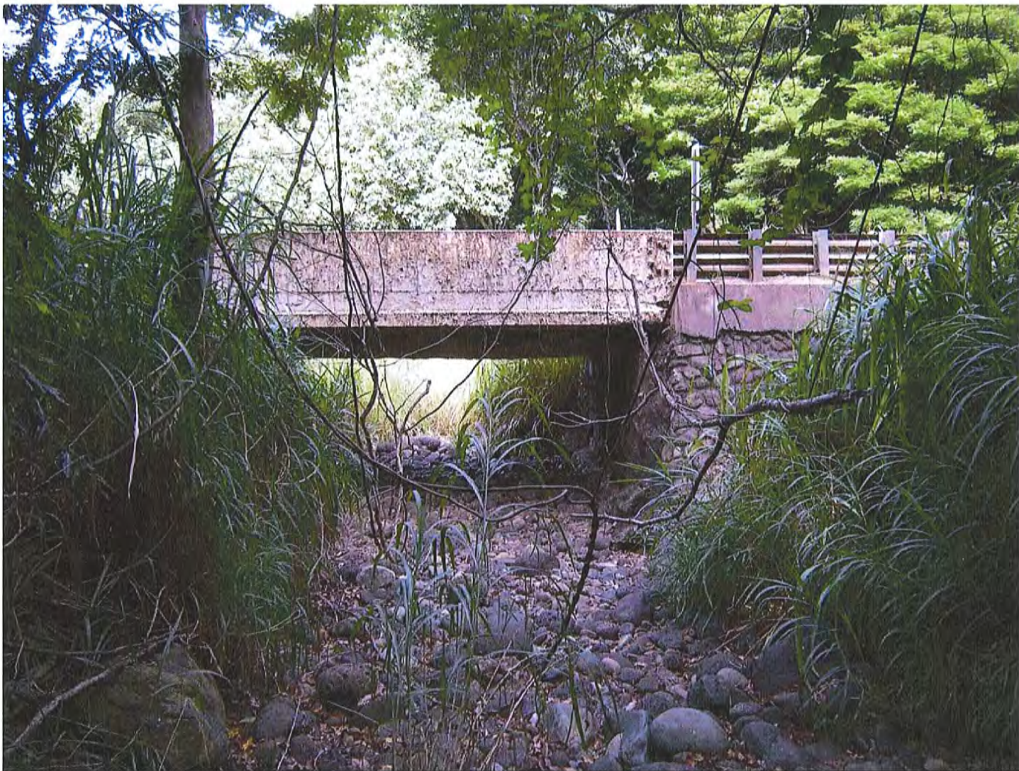
Photograph 4. HI_MauiCounty_HonoluaStreamBridge_0004. View of the bridge from the streambed on the upstream side. View facing west.
