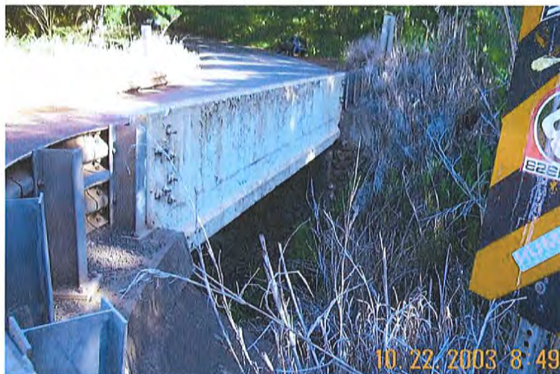
Figure 3-3. Honolua Bridge, looking at the upstream face.
