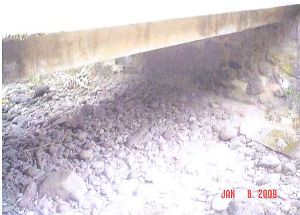
Photo 2 – Streambed under bridge structure
