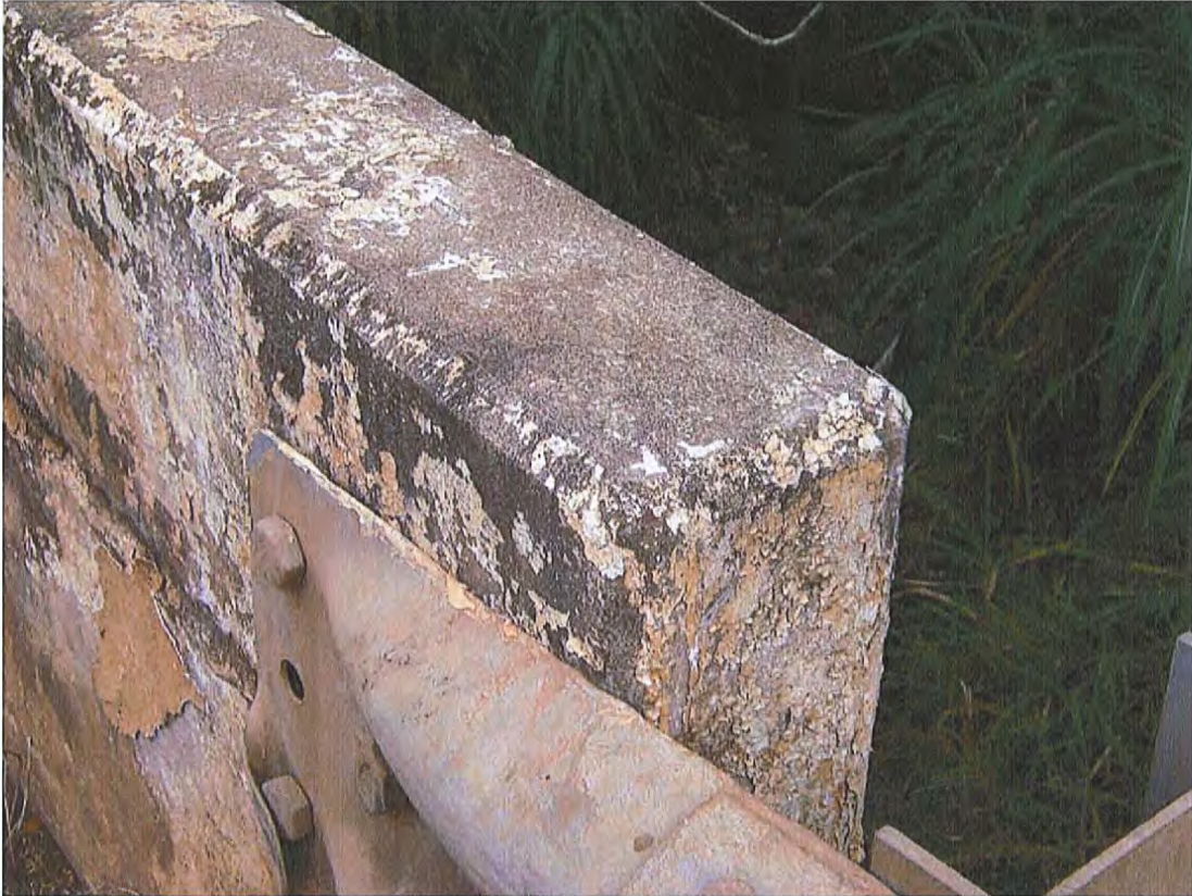
Photograph 8. HI_MauiCounty_HonoluaStreamBridge_0008. Detail of the south end of the upstream parapet showing the chamfered edges. View facing northeast.
