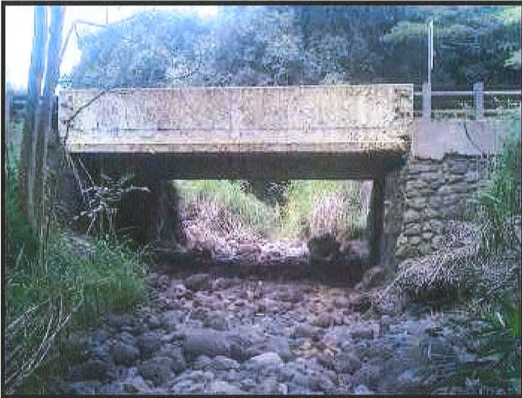
Figure 13: View East of SIHP No. -1754 Feature 11 Showing Bridge Crossing Honolulu Stream
