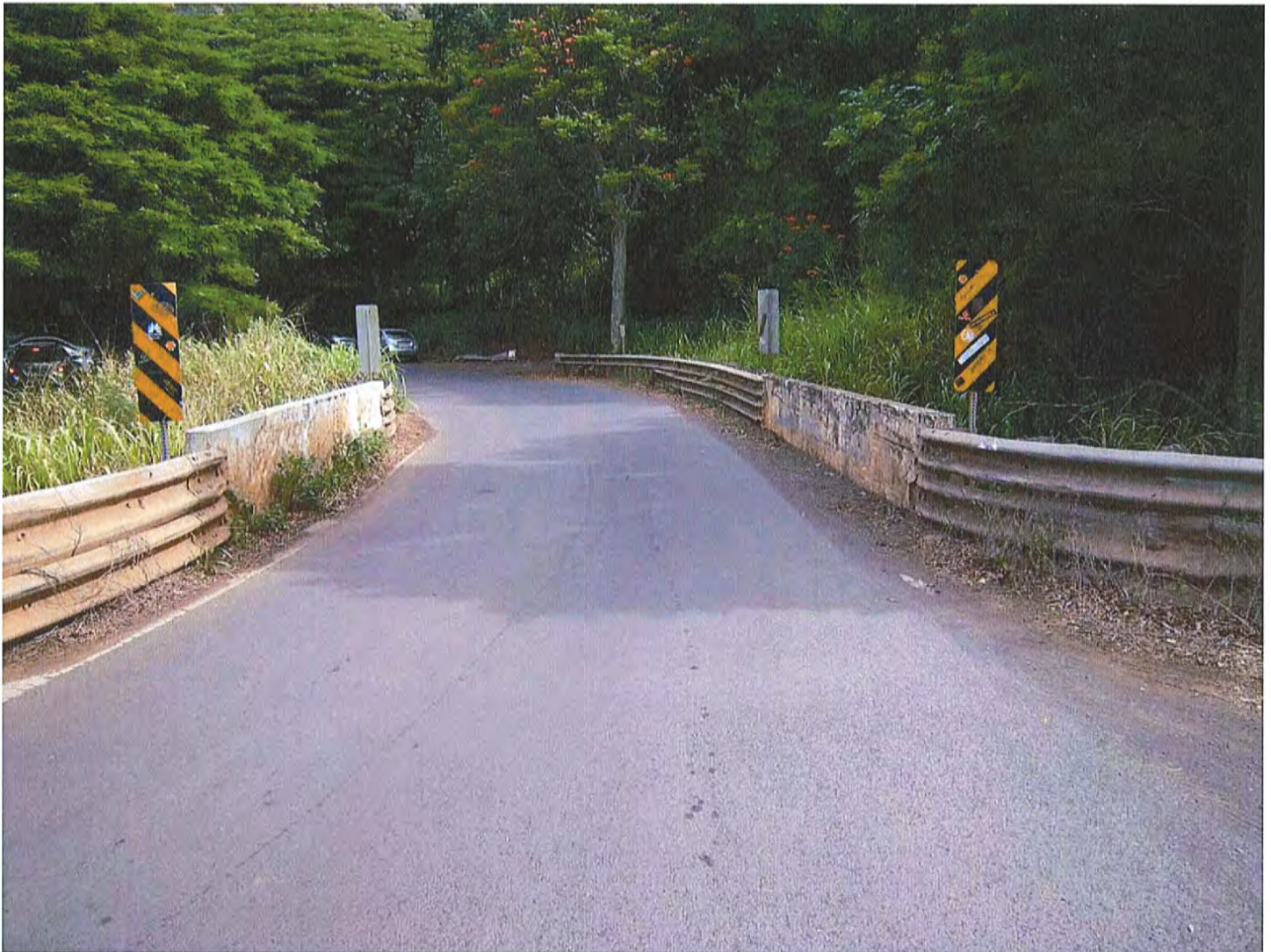
Photograph 1. HI_MauiCounty_HonoluaStreamBridge_0001. Overview of the bridge. View facing north, upstream to the right.
