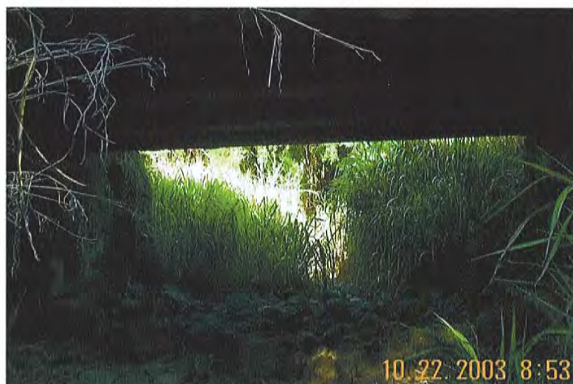
Figure 3-4. Honolua Bridge, looking upstream through the bridge.
