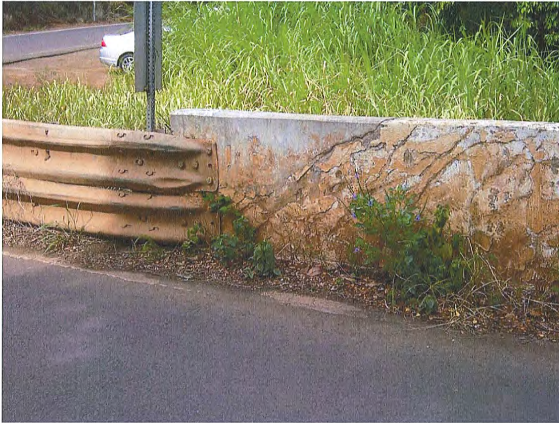
Photograph 9. HI_MauiCounty_HonoluaStreamBridge_0009. Detail of the repaired area of the downstream parapet. View facing southwest.
