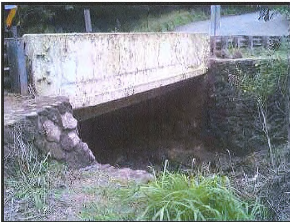
Figure 14: View South of SIHP No. -1754 Showing Bridge
