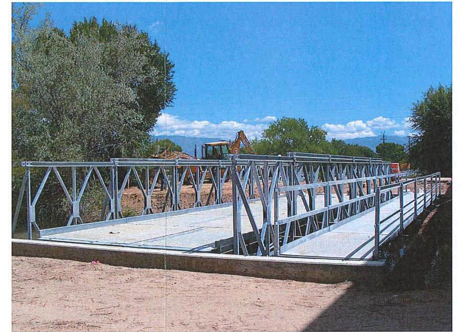
Temporary Bridge and Pedestrian Walkway
