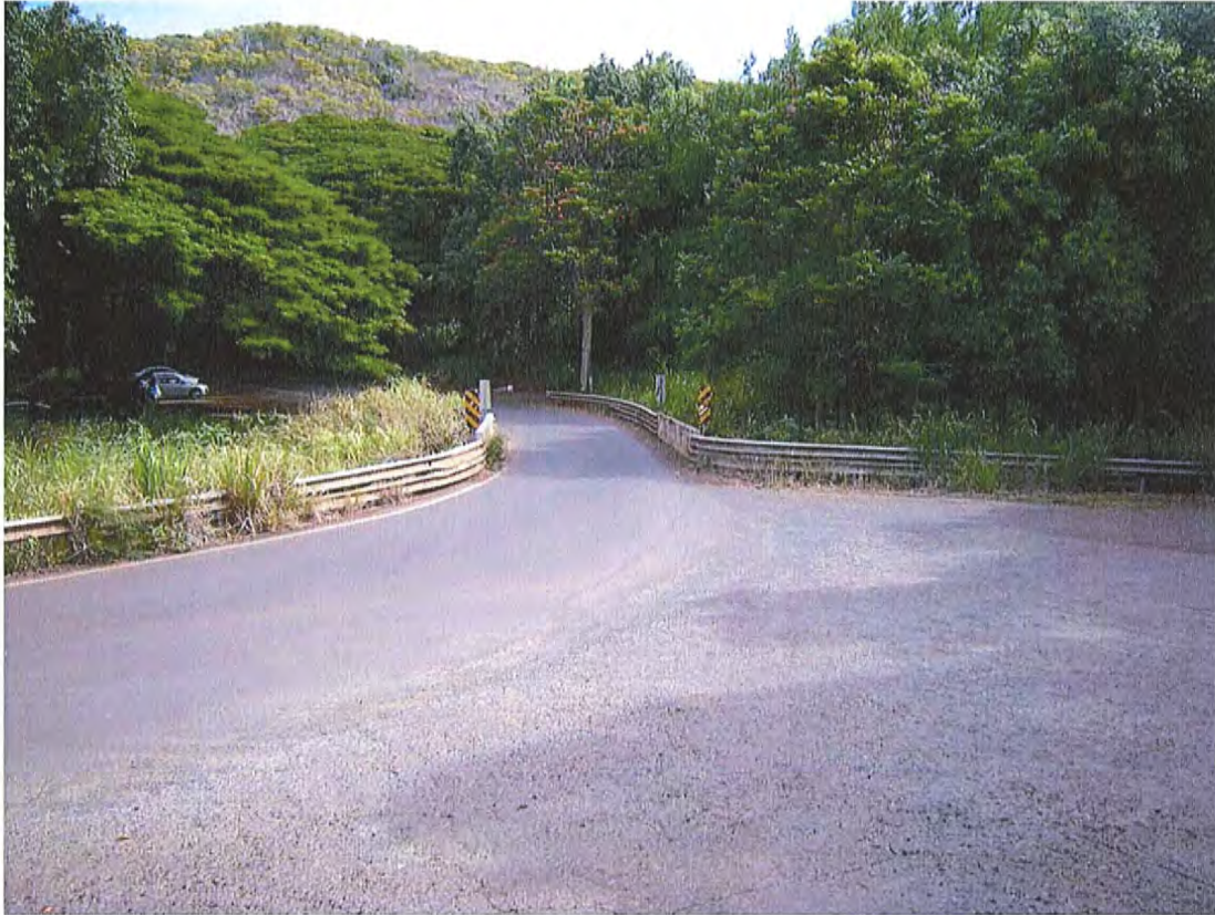
Photograph 3. HI_MauiCounty_HonoluaStreamBridge_0003. Wide overview of the bridge showing the rural setting with a parking area in the left background. View facing north.
