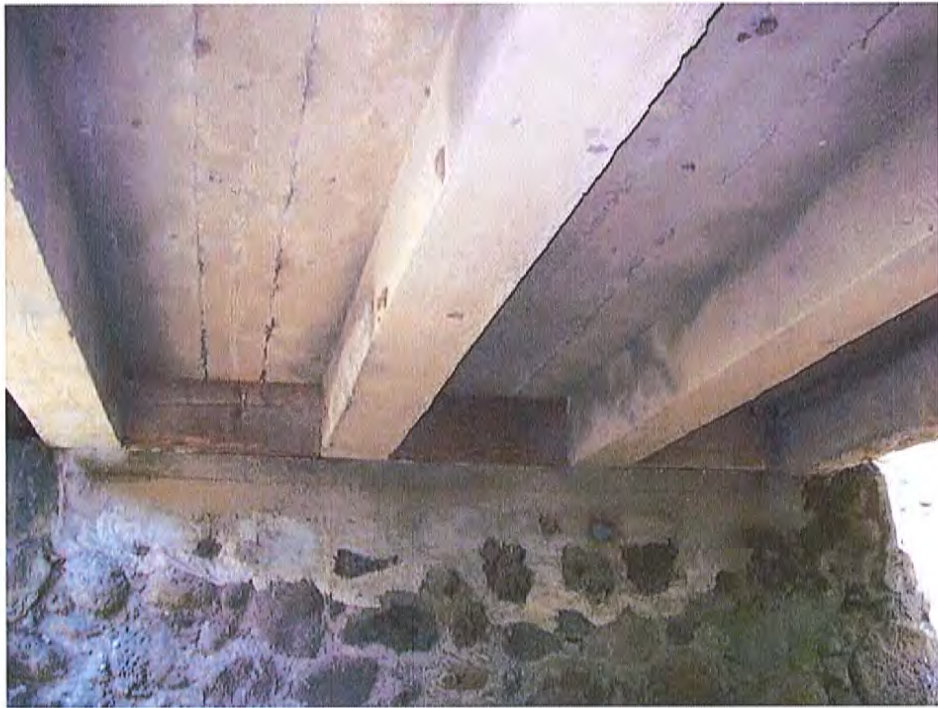
Photo 4 – Underside of bridge
