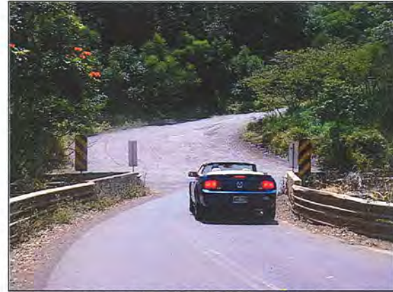
Figure 3. Photograph of the Honolua Stream Bridge. (Photo courtesy of HHDOT.)
