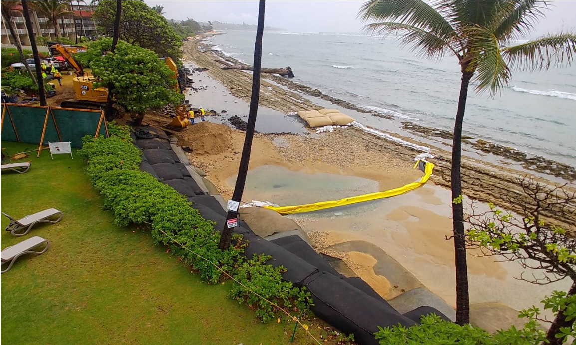
Figure 22. Photograph taken on March 23, 2023, at 9:33 AM, during project construction
