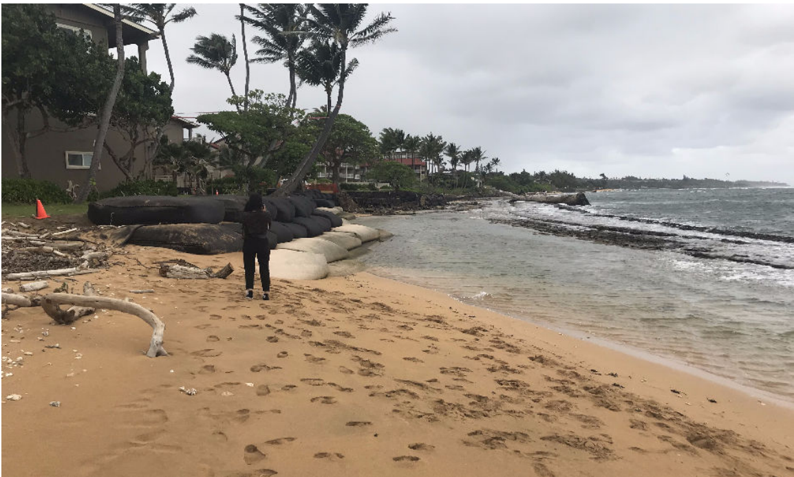
Figure 4. Photograph taken before construction, on January 18, 2021, showing southern end of pre-existing sandbag shoreline protection fronting the Condominiums, facing north
