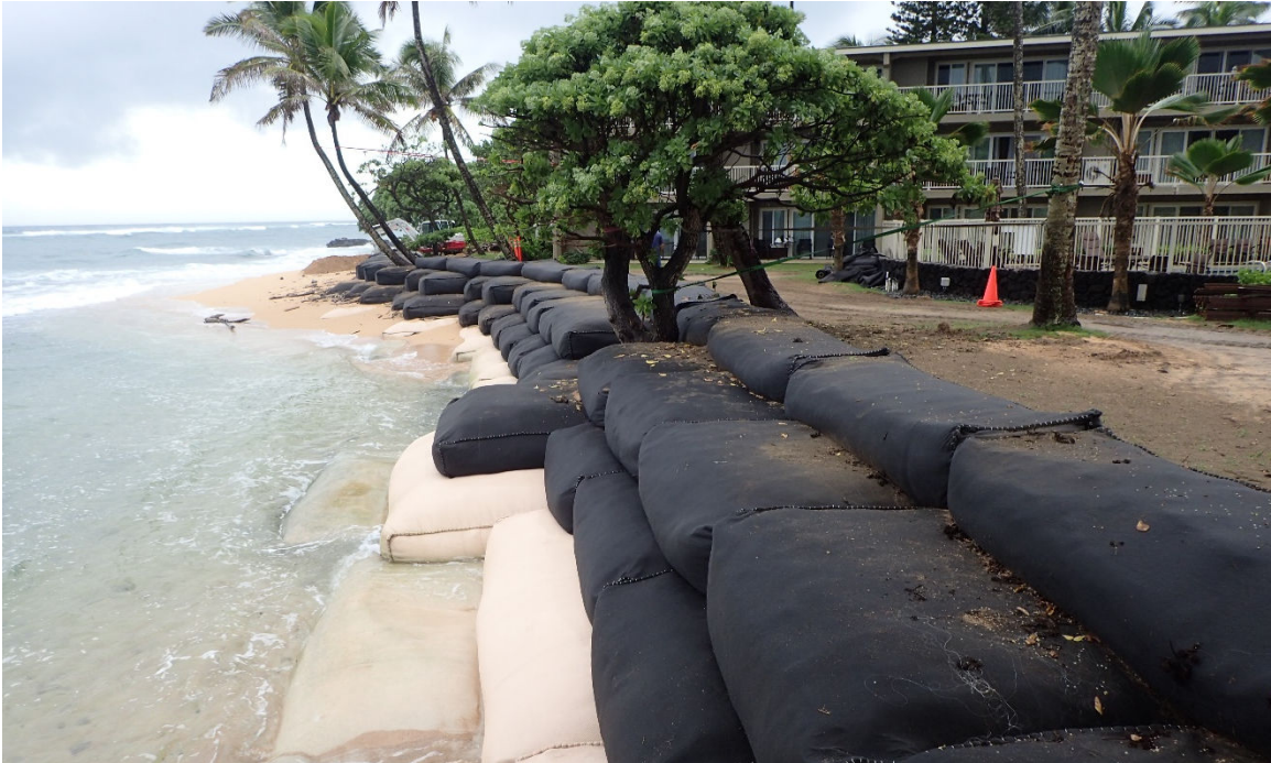
Figure 3. Photograph taken before construction, on October 20, 2020, showing pre-existing sandbag shoreline protection fronting the Condominiums, facing south
