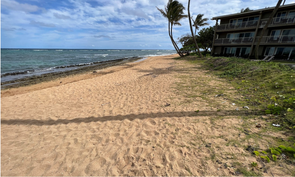
Figure 17. Photograph taken after vegetation establishment, on March 19, 2024, showing beach nourishment and vegetated sand berm, facing south
