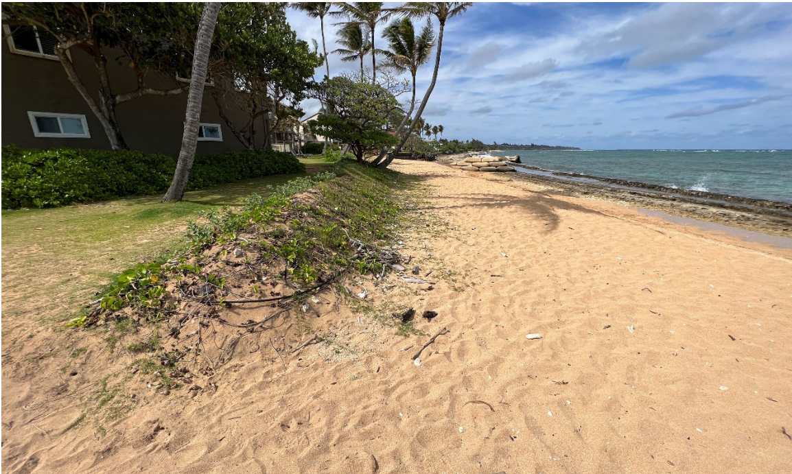
Figure 18. Photograph taken after vegetation establishment, on March 19, 2024, showing sandbag groin, beach nourishment and vegetated sand berm, facing north
