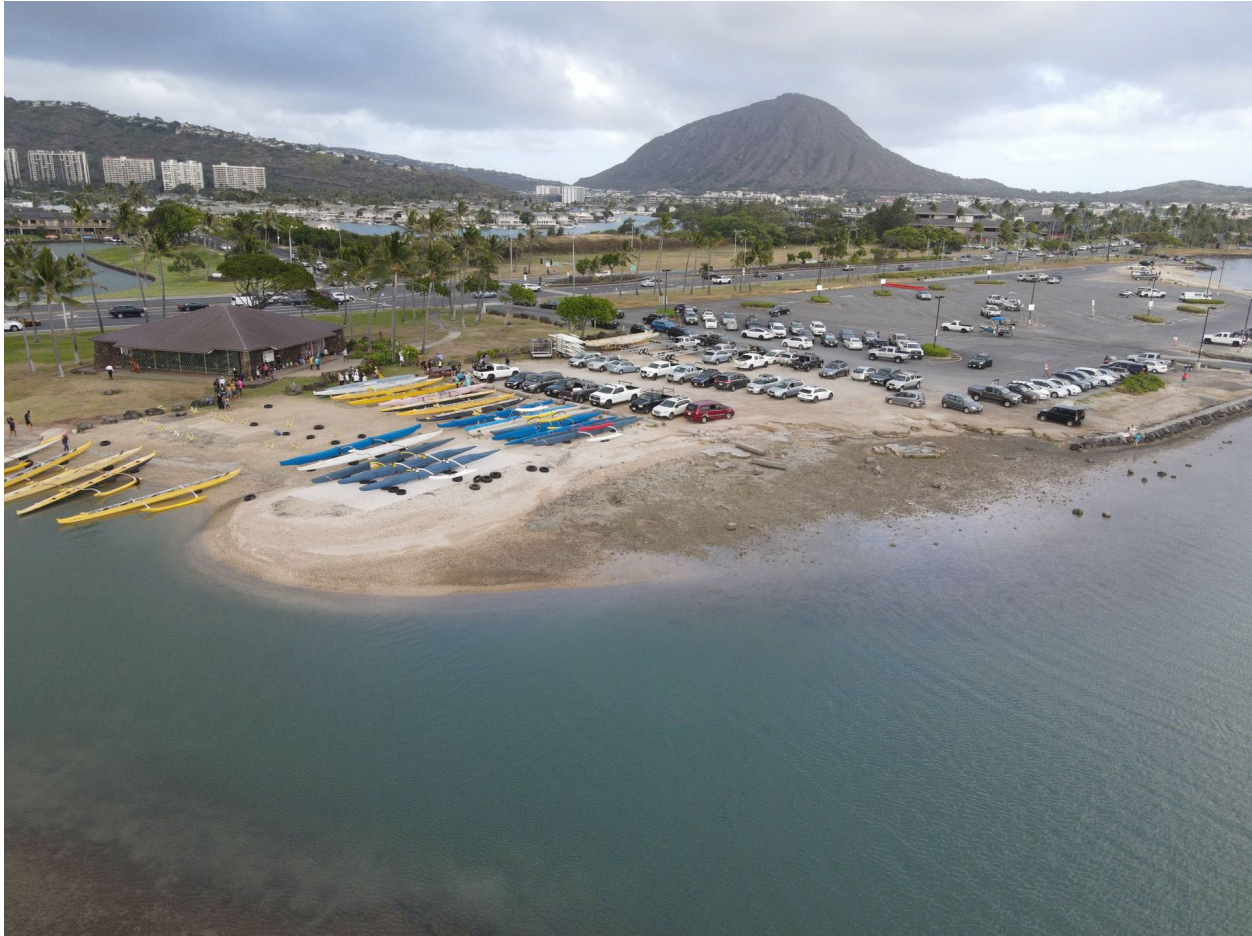
Figure 4. Oblique Aerial Photograph of the West End of the Facility as It Existed on April 13, 2022 (Photo: Shoreline Science & Engineering, LLC)
