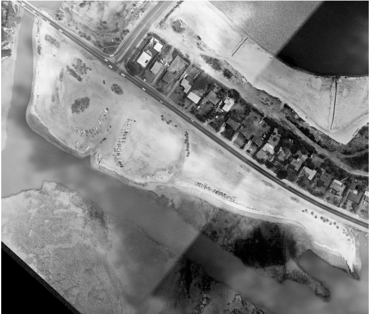
Photograph 2, the facility as it existed shortly after its original construction as shown in an aerial photograph captured in 1967.
