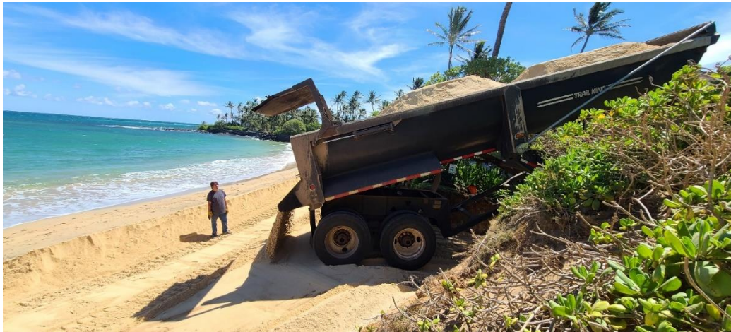
Figure 6-1. Dump truck delivering sand to the west end of the cove for placement on the berm (Maintenance #3)
