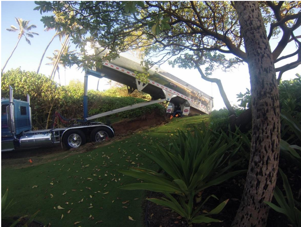
Figure 4-1. Sand delivery to the west end of the cove for placement on the berm (Maintenance #1)
