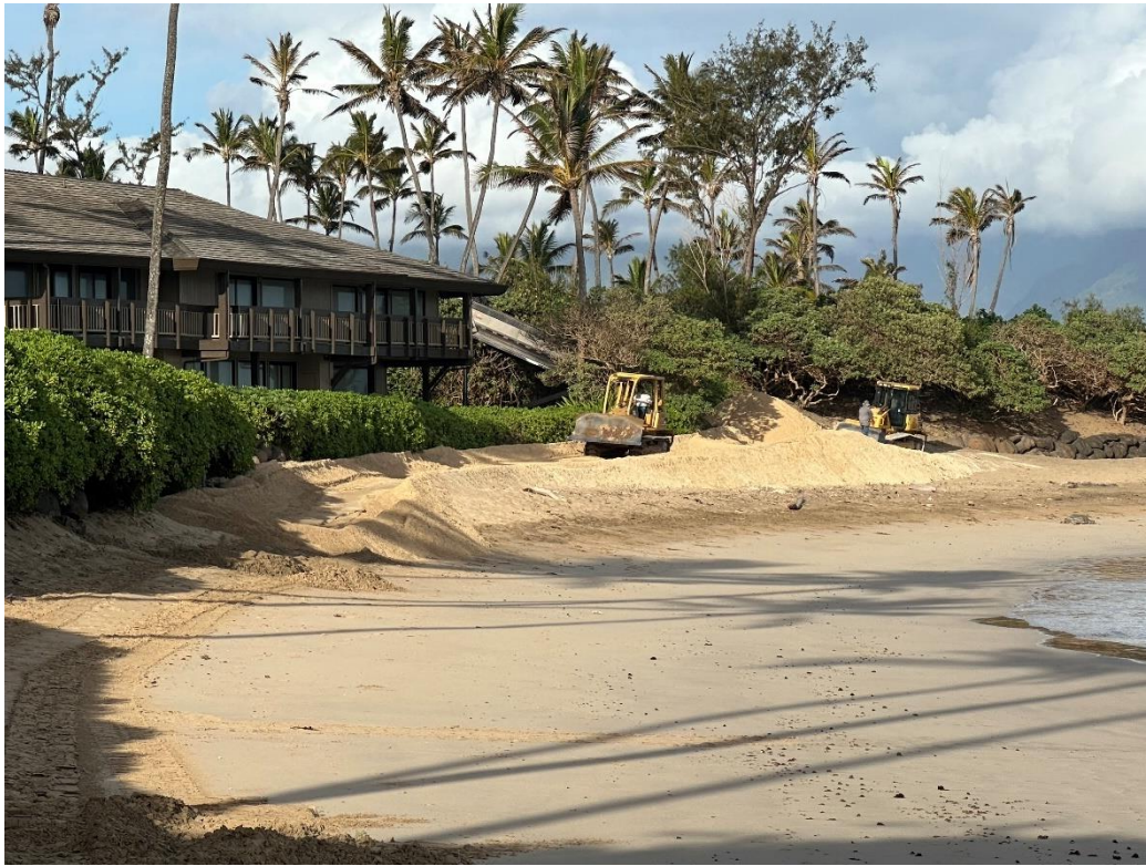
Figure 8-1. Dump truck delivering sand to the west end of the cove for placement and bulldozers spreading sand on the berm (Maintenance #5)
