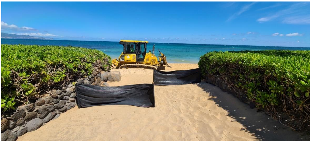
Figure 6-2. Bulldozer spreading sand along the berm (Maintenance #3)
