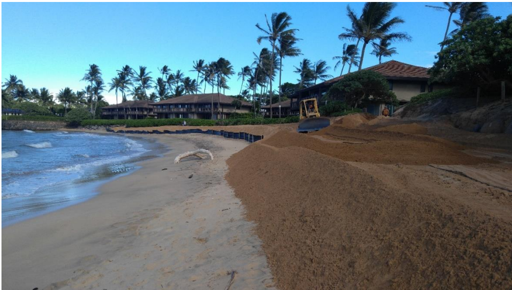
Figure 5-2. Bulldozer spreading sand along the berm (Maintenance #2)
