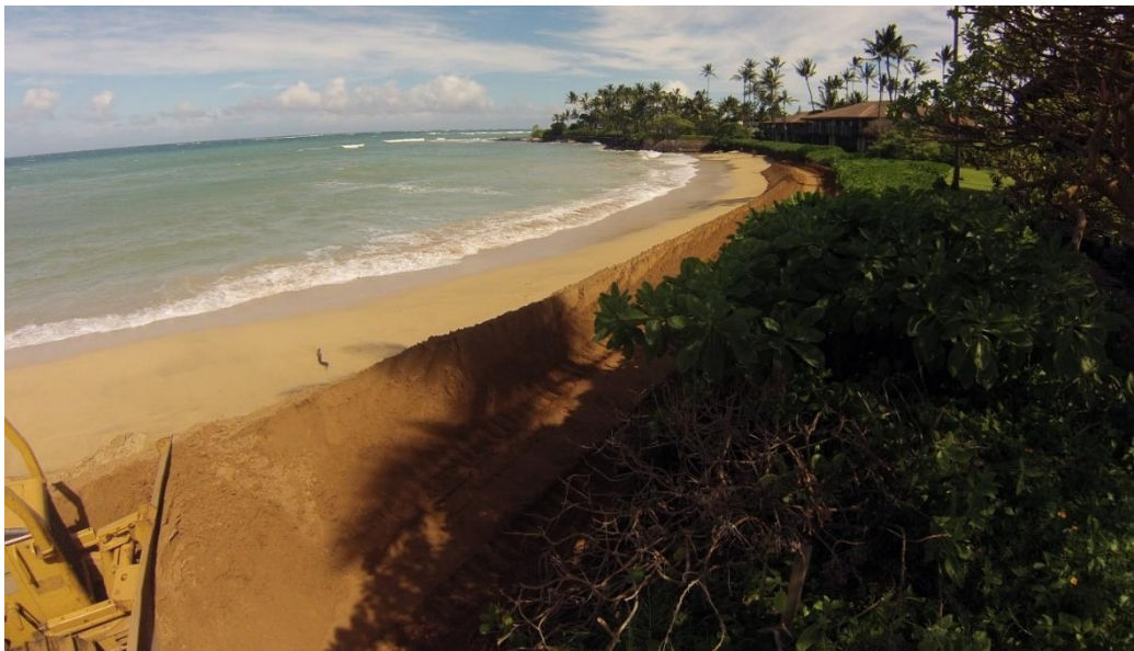
Figure 4-4. Sand grading on the berm (Maintenance #1)
