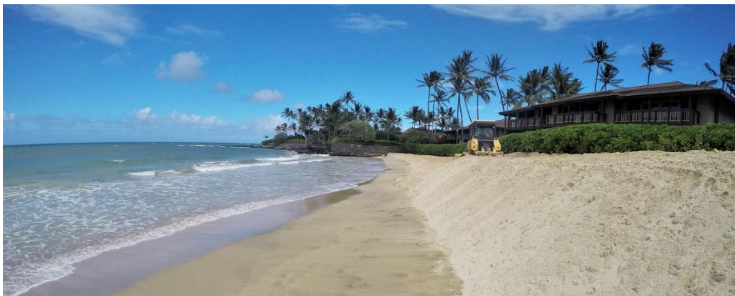
Figure 7-3. Graded sand with finished makai slope ending near the public access at the eastern neighbor's seawall (Maintenance #4)
