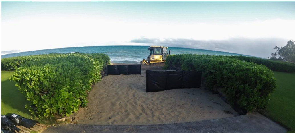
Figure 7-2. Bulldozer spreading sand along the berm (Maintenance #4)
