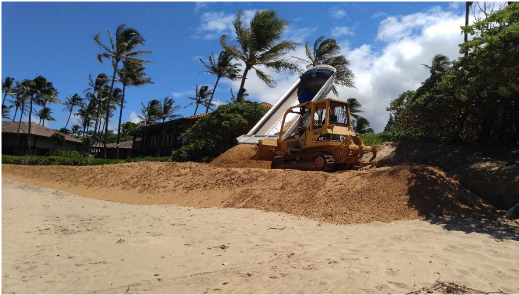
Figure 5-1. Dump truck delivering sand to the west end of the cove for placement on the berm (Maintenance #2)
