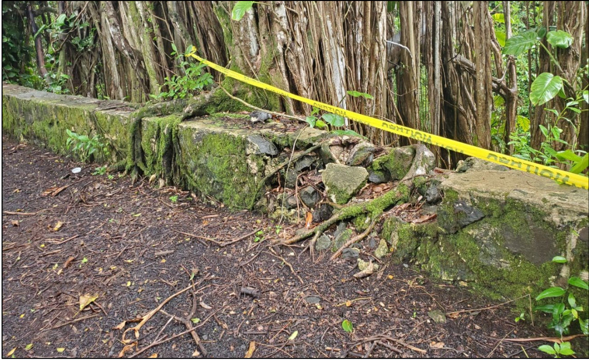
Photo 3. Small section of CRM wall damaged by Chinese banyan tree roots.
