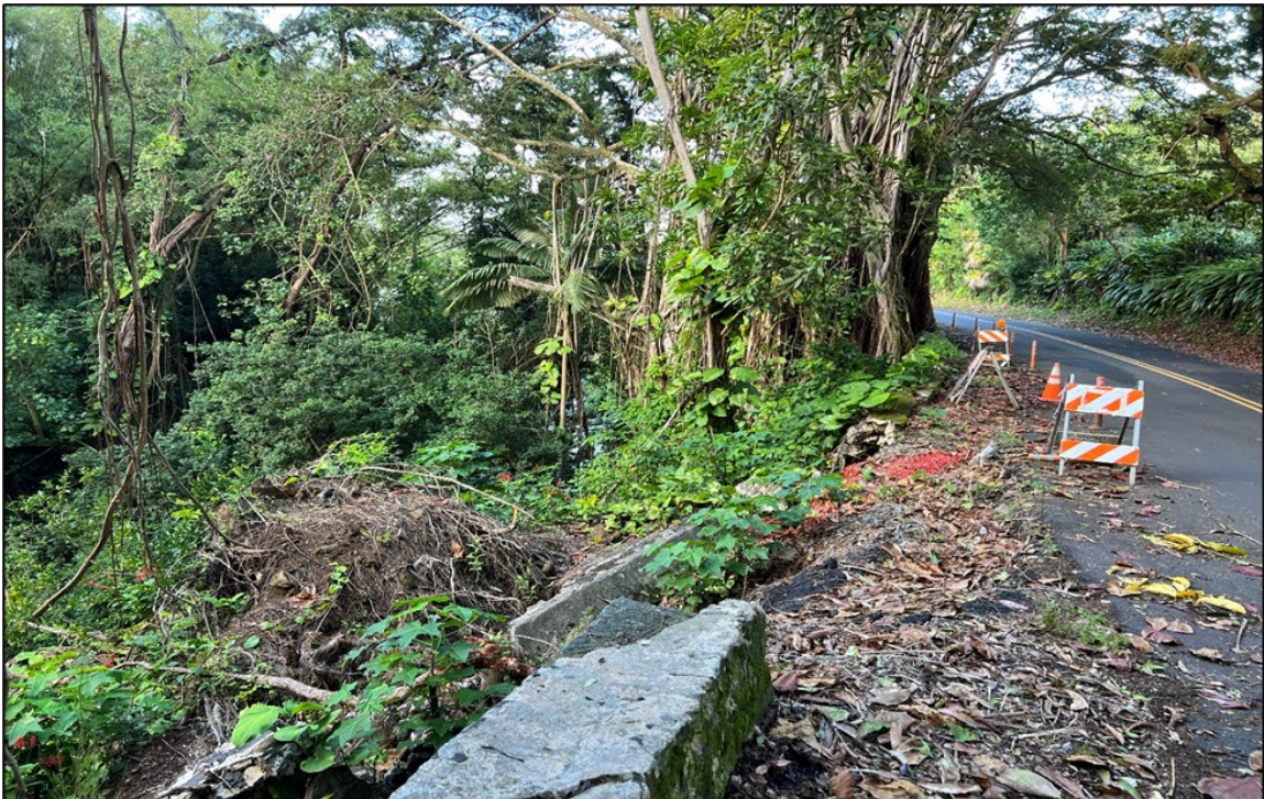
Photo 2. Uprooted Chinese banyan tree tree that damaged an approximately 55-foot-long section of CMR wall, view looking west.
