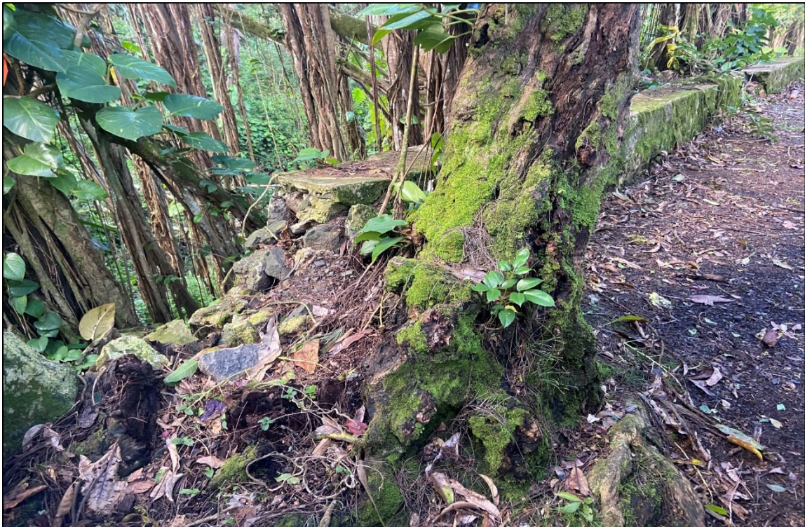
Photo 4. Small section of CRM wall damaged by Chinese banyan tree roots and an ironwood tree growing on the roadway side of the CRM wall.
