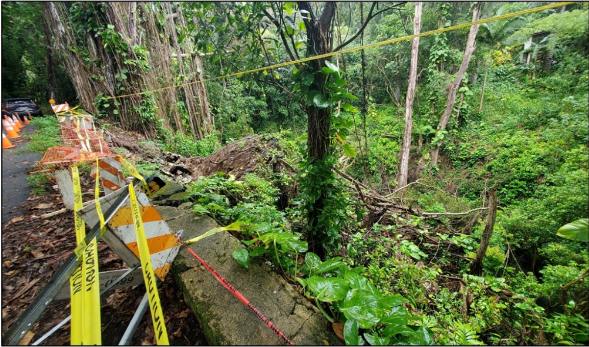
Photo 1. Uprooted Chinese banyan tree that damaged an approximately 55-foot-long section of CMR wall, view looking east.
