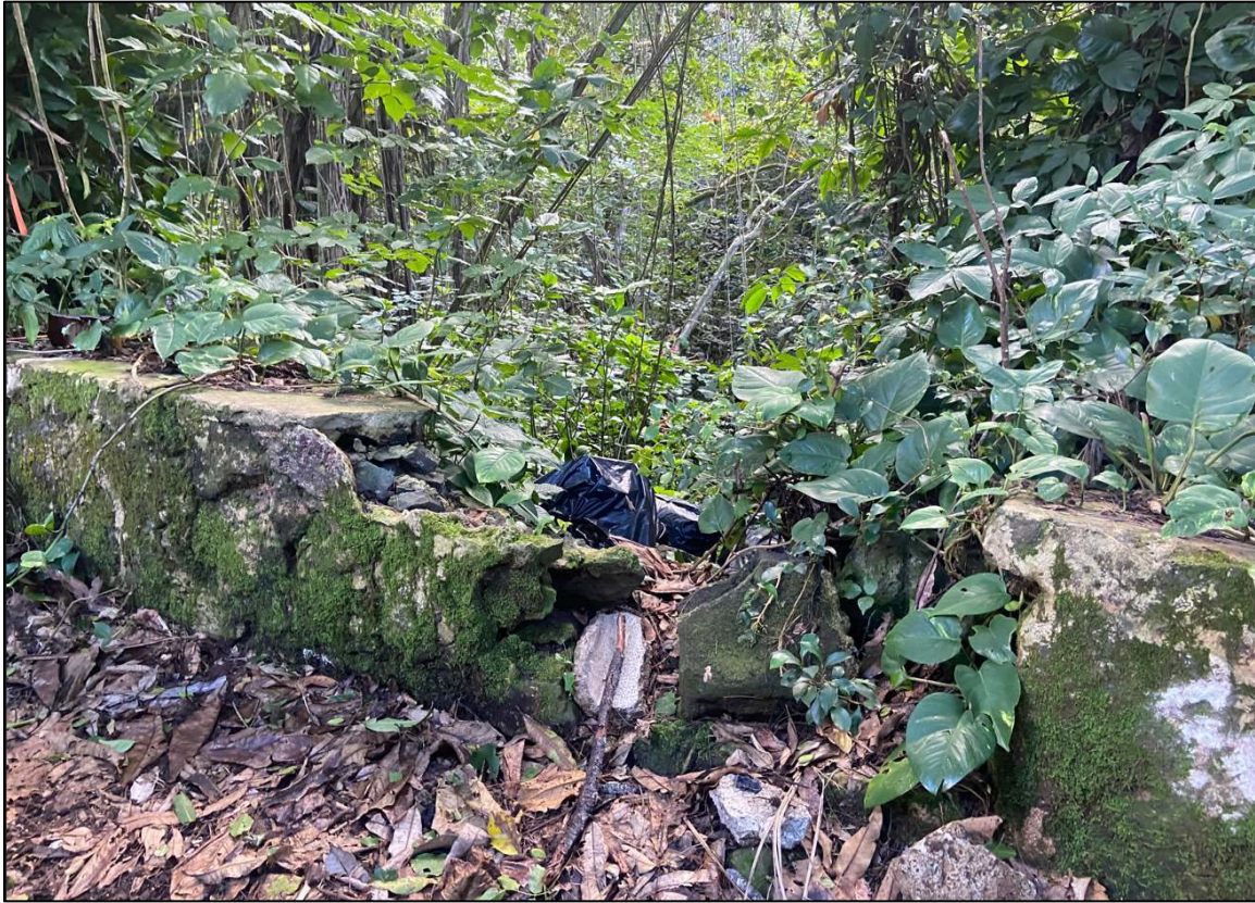
Photo 5. Small section of damaged CRM wall.
