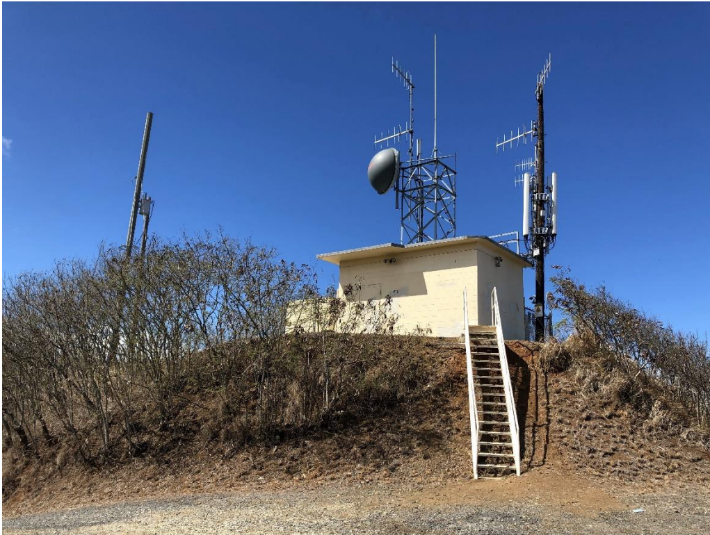
Figure 3: Building North View (T-Mobile compound behind HECO building. T-Mobile's existing antennas visible on the wood utility pole on the right of building.)
