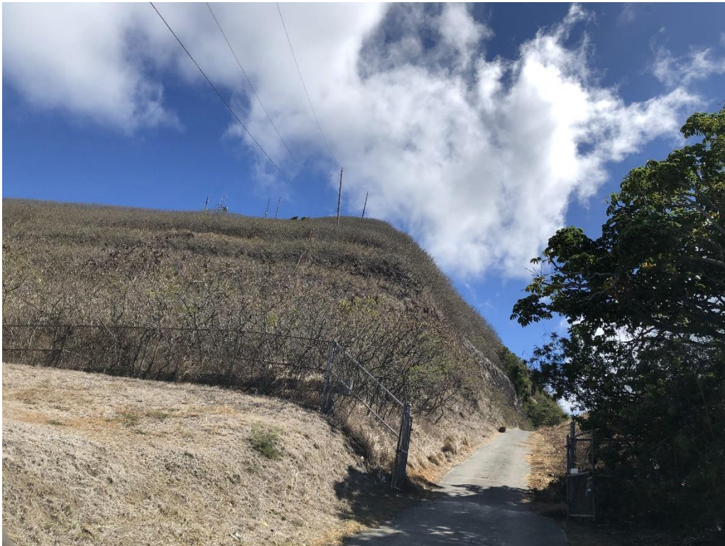
Figure 2: Access road with gate open
