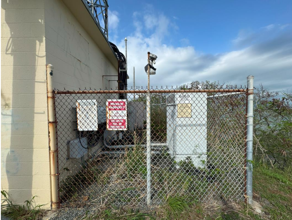
Figure 5: T-Mobile compound West View
