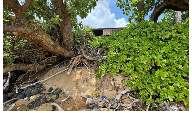
Photograph 2. Fronting the property of TMK 4-3-009:026, looking west at the property
