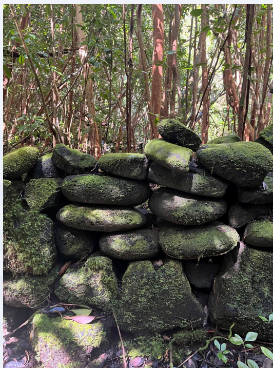
Figure 34. Historic rock wall along the Puna Trail, featuring the traditional 'alā stones used in construction of the ala loa.
