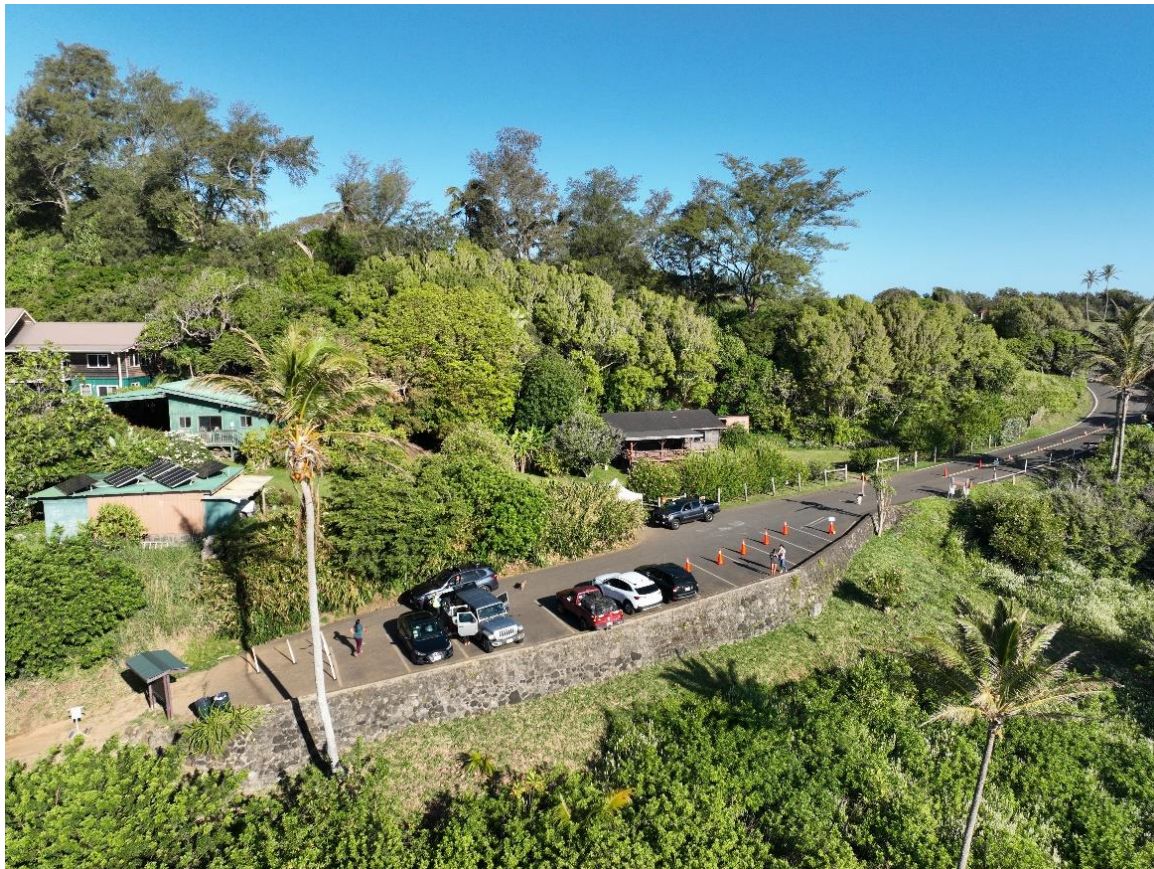
Current parking/lookout area envisioned to be re-designated for cultural/special access.
