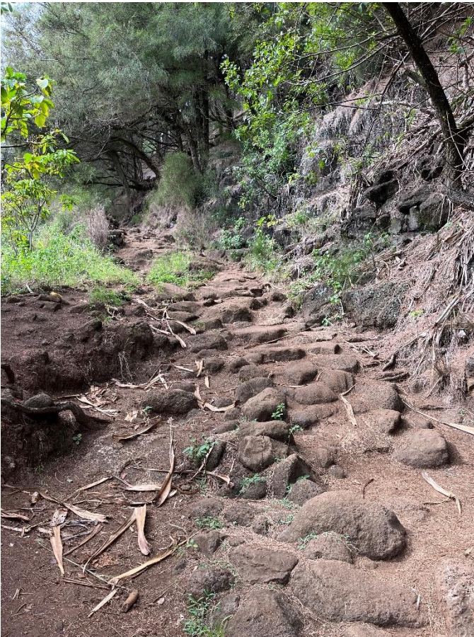
(Top) Historic retaining wall along the trail; (Bottom) Historic cobble stones embedded in sections of the trail.
