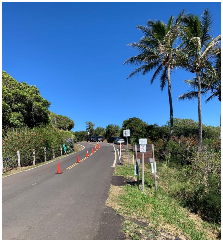
View (from the trailhead) of 'Akoni Pule Highway under the jurisdiction of the County Department of Public Works.
