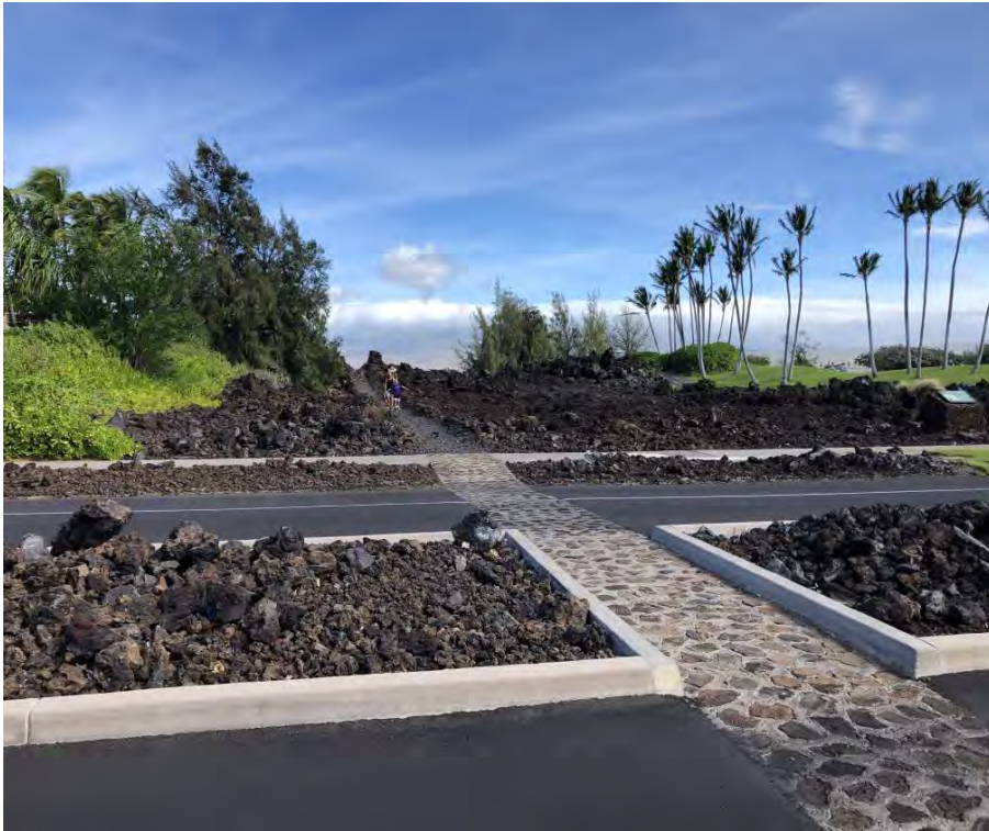
← This is the recommended breach surface treatment. It resembles the authentic historic surface while enabling road use. Photo taken in Waikoloa Resort
