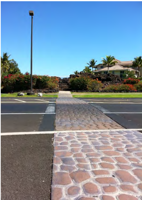
← The reddish, smooth cobblestone appearance of this surface treatment is artificial and does not resemble any historic Hawaiian trail surface. Photo taken in Waikoloa Resort
