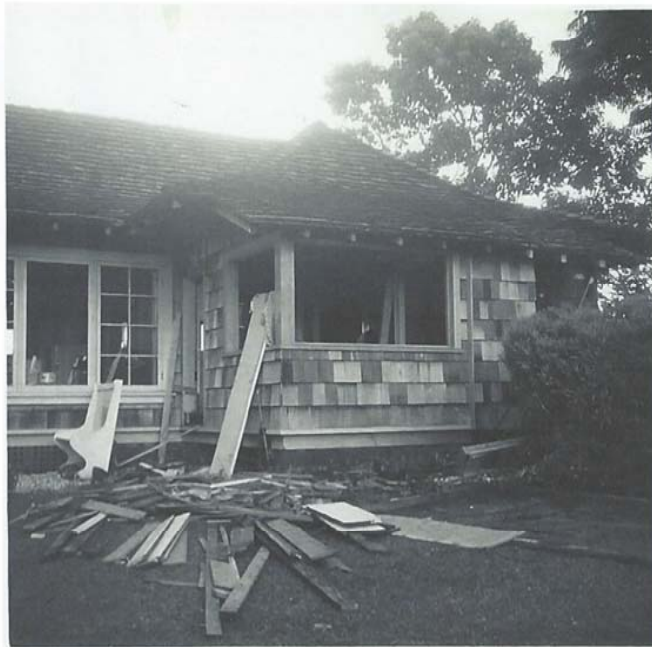
PHOTO 41: 1954 photo of the renovation/alteration of the existing house replacing the original board-and-batten exterior wall finish with wood shingle lap siding, and window replacements; note the area of construction is about the existing Kitchen and Living Room area.
