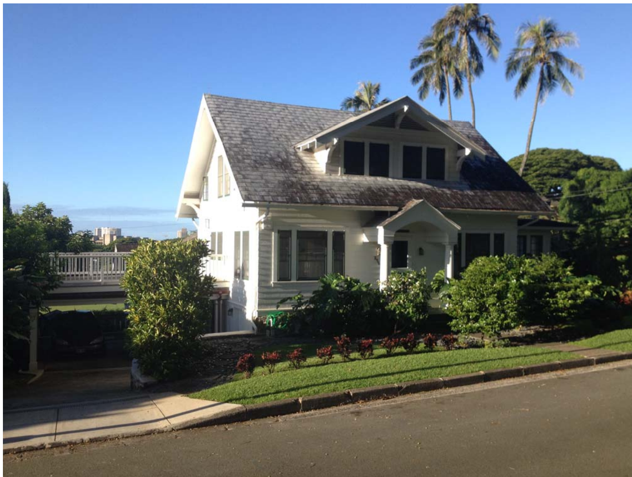
3 of 7. Northeast elevation (front façade). Looking northwest. HI_Honolulu_Malama Manor_0003.tif
