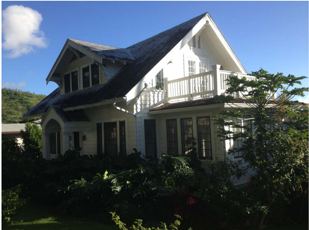
4 of 7. Northeast and southeast elevations. Looking northwest. HI_Honolulu_Malama Manor_0004.tif
