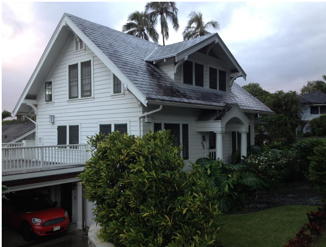
2 of 7. Northeast and southeast elevations. Looking northwest. HI_Honolulu_Malama Manor_0002.tif
