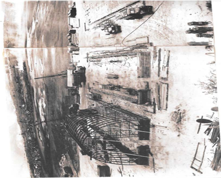
Fig. 5a – Quonset Hut being assembled in the Waiawa Gulch consist of buildings in a semi-urban Industrial setting
