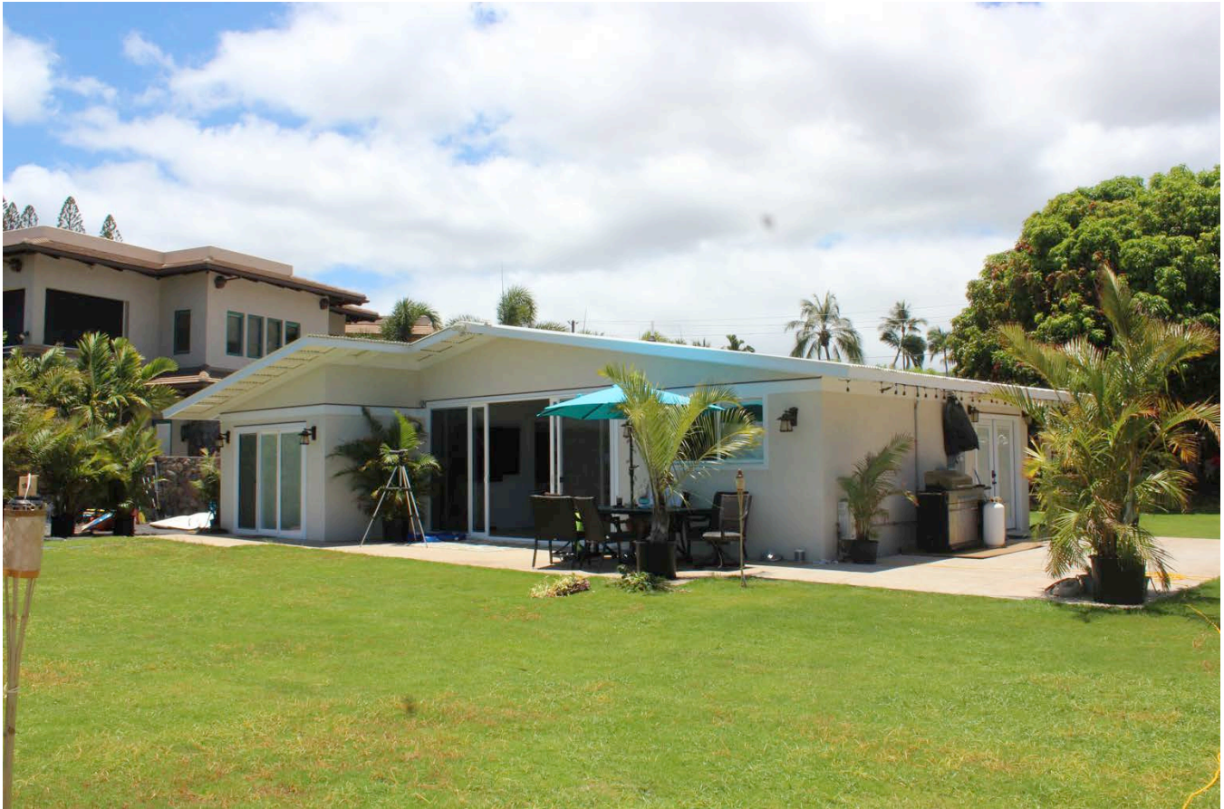
Photo 006 (HI_Maui_MaryPBrightHouse_006). Mary P. Bright House, oblique view of rear (Southwest) facade, camera facing Northwest.
