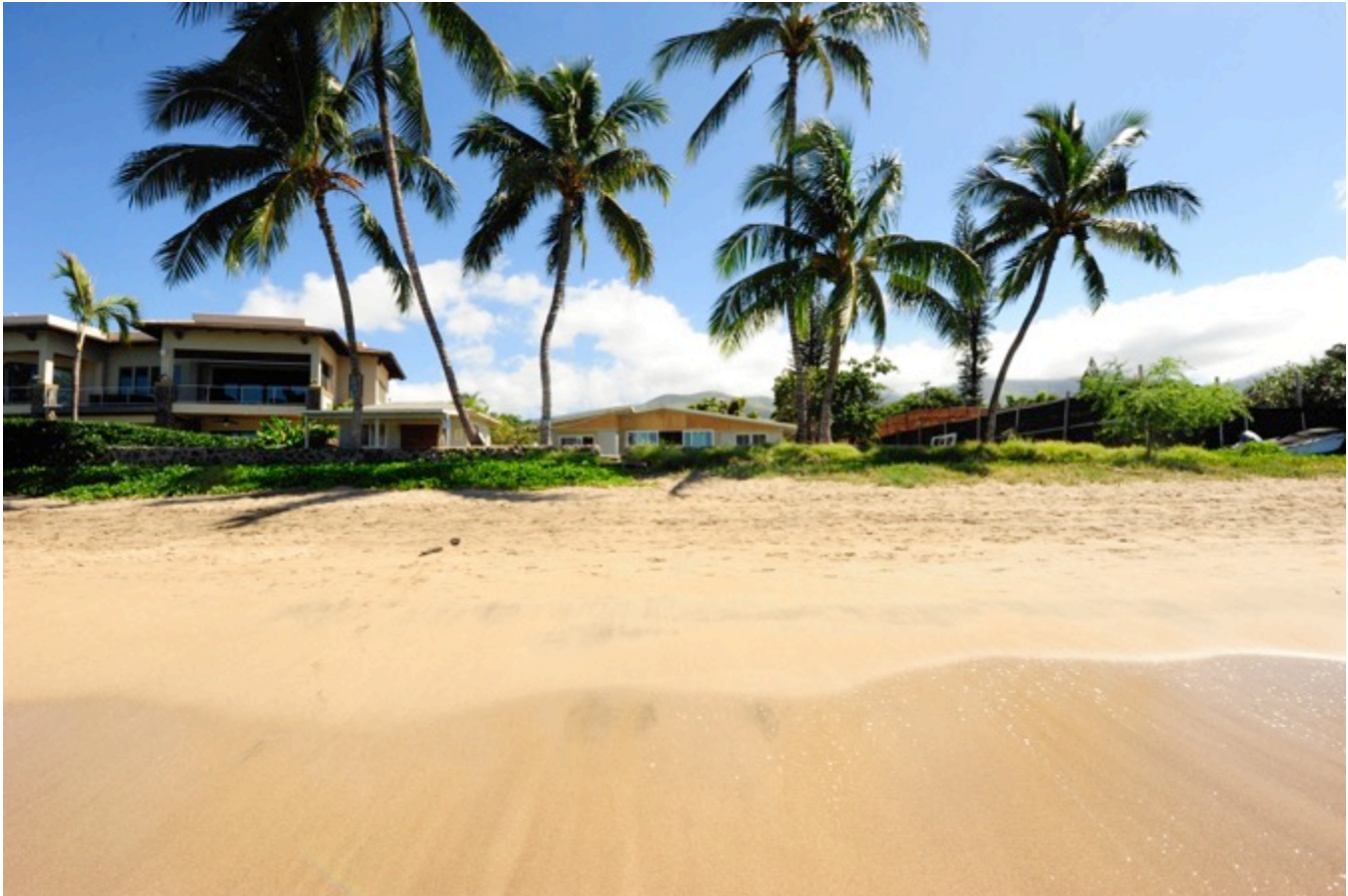
Photo 004 (HI_Maui_MaryPBrightHouse_004) Mary P. Bright House, view of rear (Southwest) facade, camera facing Northeast
