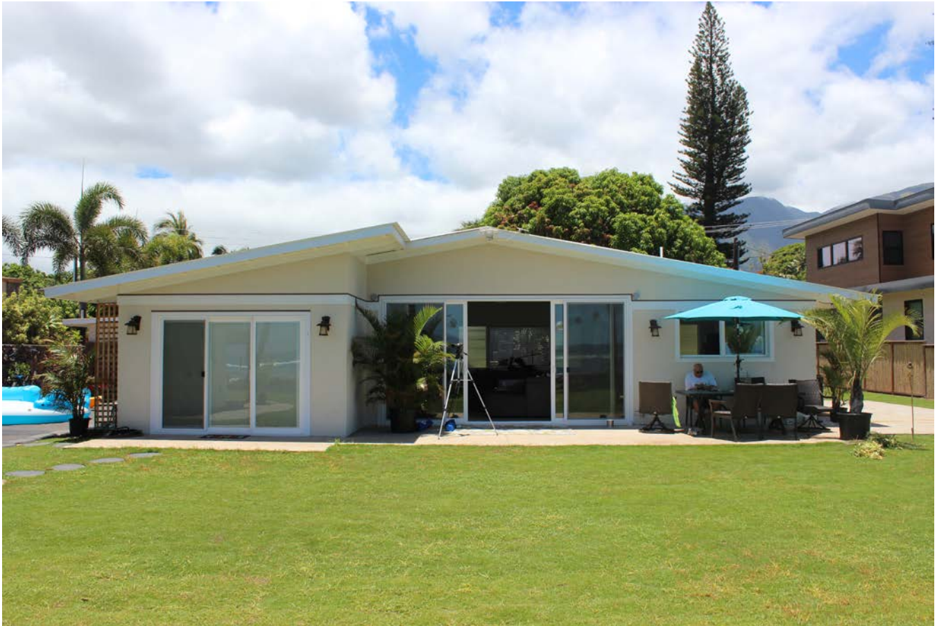
Photo 005 (HI_Maui_MaryPBrightHouse_005) Mary P. Bright House, detail view of rear (Southwest) facade, camera facing Northeast
