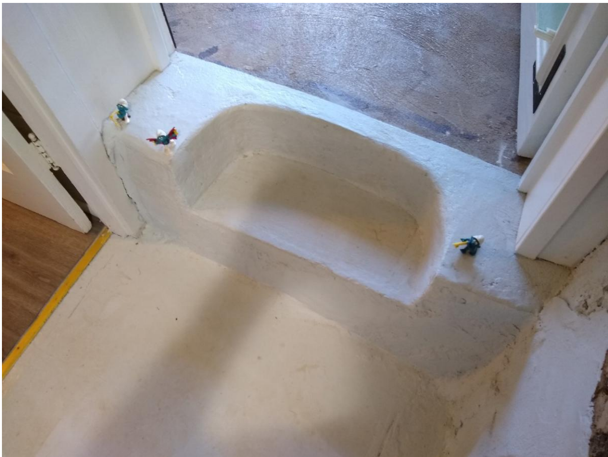
Cast Concrete step from Garage to forward storage area, Lower Level
