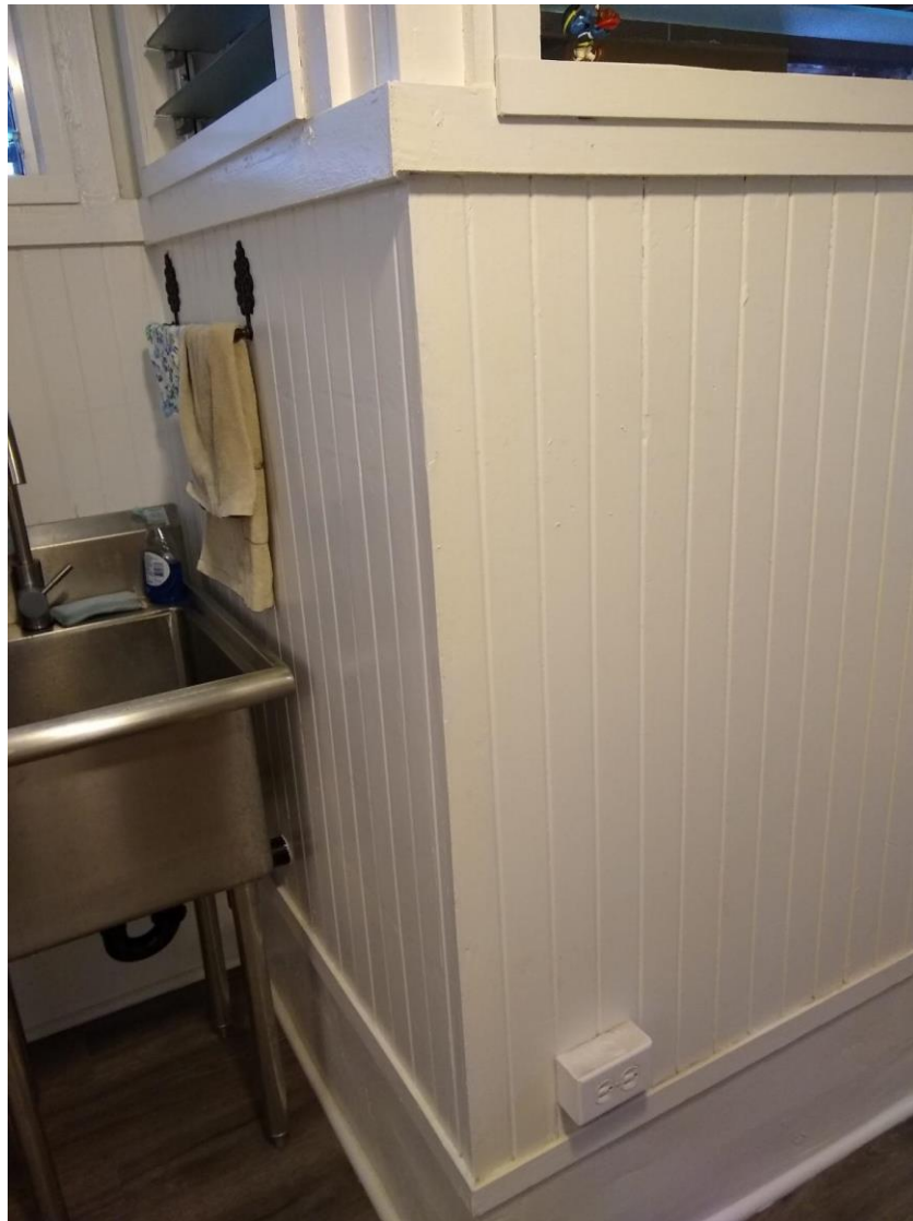
Bead-board Wainscot of lower level, eastern wall
