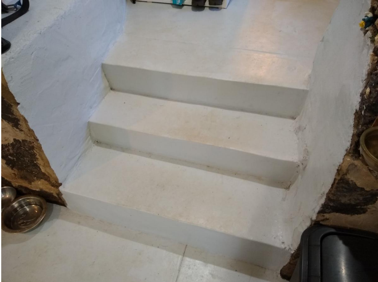
Cast Concrete Steps from the Garage to the Mud Room
