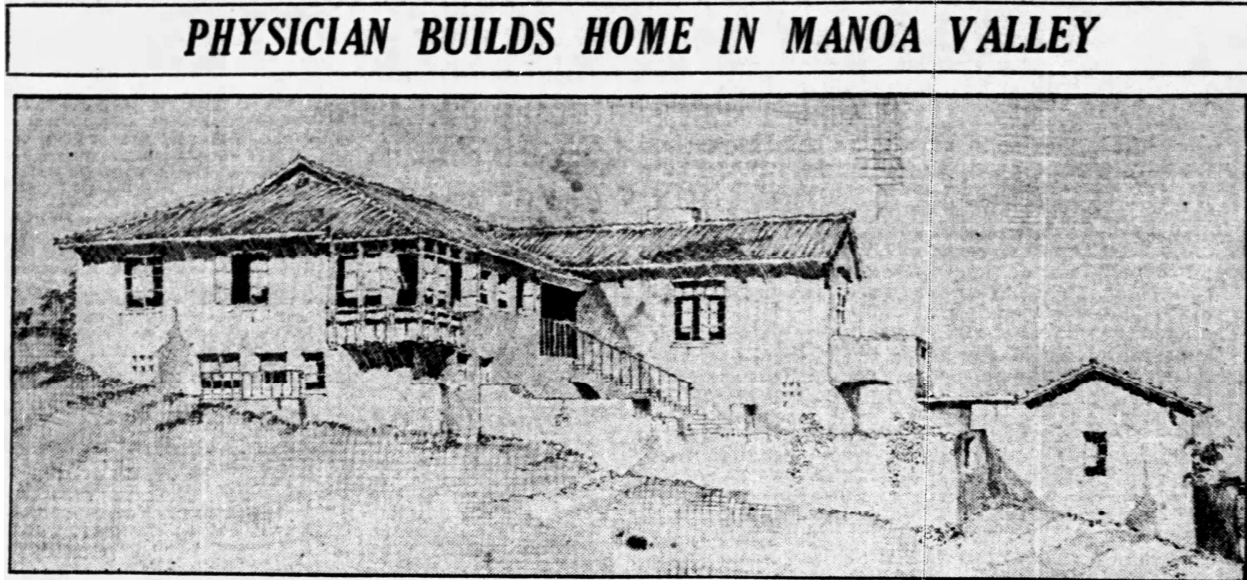
This residence is in the process of construction near the Dr. Paul Withington home in Upper Manoa valley. It is for Dr. V. E. M. Osorio. Cost of construction will approximate $17,000. Architectural work was done by the firm of Robert Miller.
