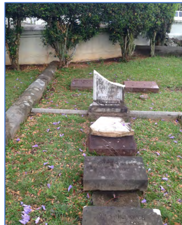
Left and right: Kawaiaha'o flawed stones that cracked as a result of weathering and moisture seeping into those flaws. These stones have slotted pedestals.
