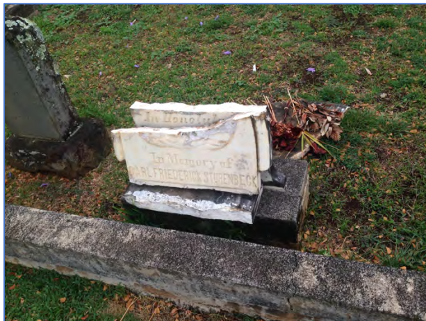
Left and right: Kawaiaha'o flawed stones that cracked as a result of weathering and moisture seeping into those flaws. These stones have slotted pedestals.
