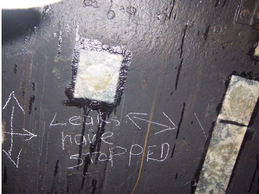
Re-patched holes in bulkheads in Tank #4 port.
