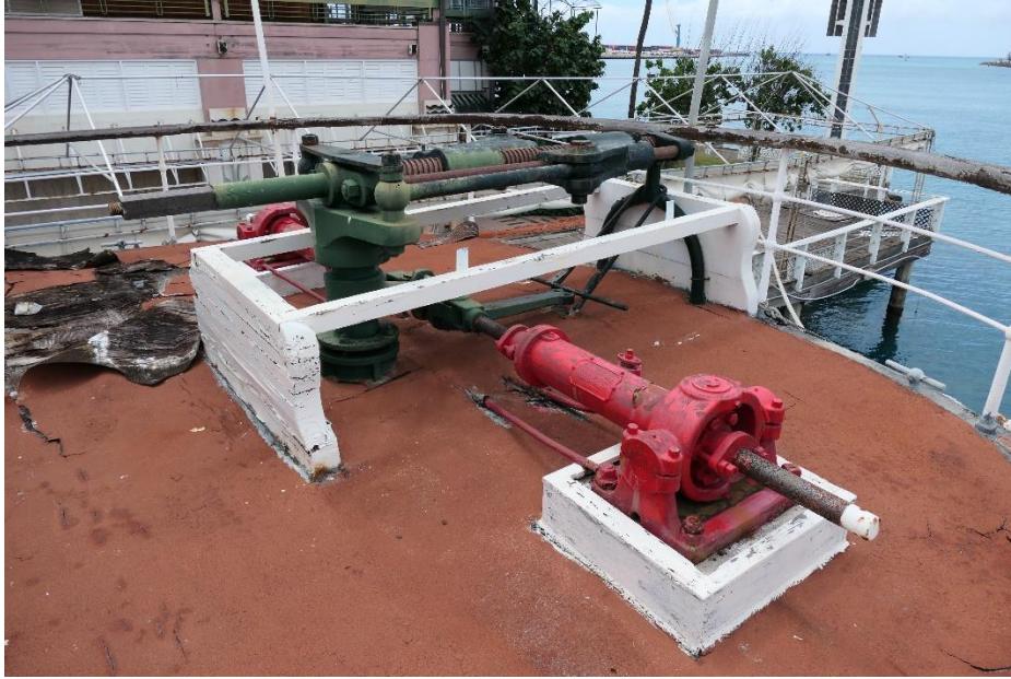
Figure 21: The Krough Manufacturing Co. steering apparatus on the decayed, collapsing poop deck (Joseph Lombardi).
