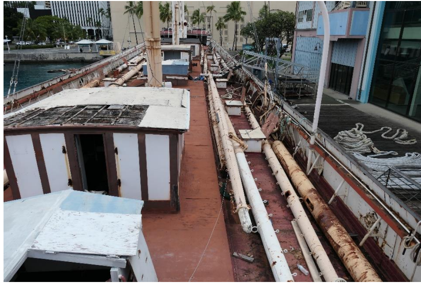
Figure 18: The corroding, dry-rotted and crowded decks of the ship are in danger of collapse and a hazard to anyone who boards the vessel (Joseph Lombardi).
