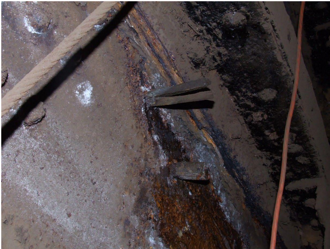
Wooden plugs keeping the ocean out.
