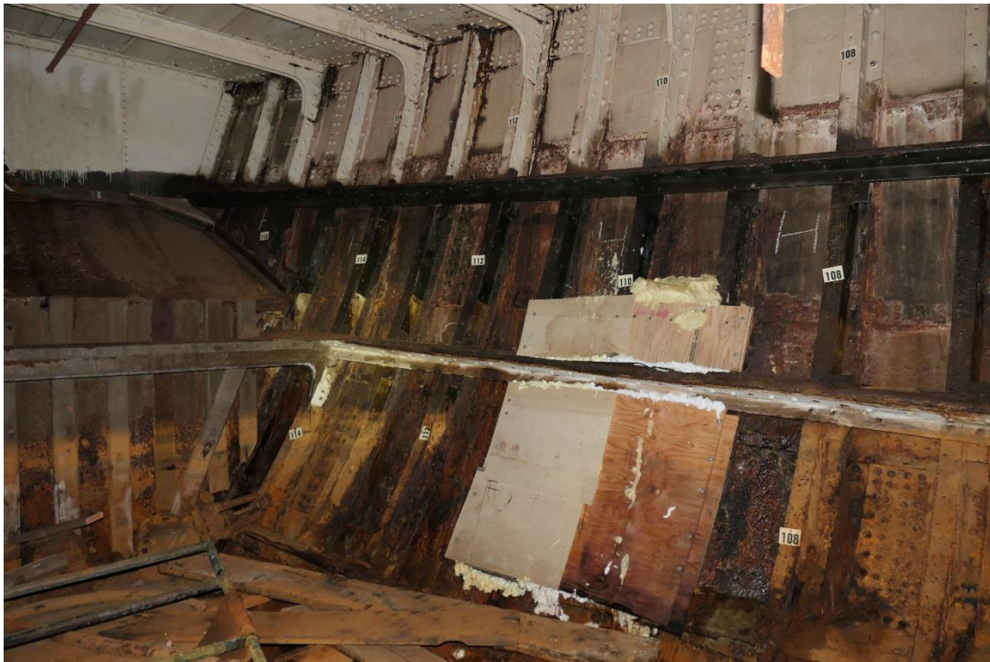
Figure 8: Larger patches cover area where the hull is leaking more substantially, but the loss of up to fifty percent of hull plating thickness in many areas, lost rivets, and rainwater entering through the decks have essentially made Falls of Clyde a floating wreck (Joseph Lombardi).
