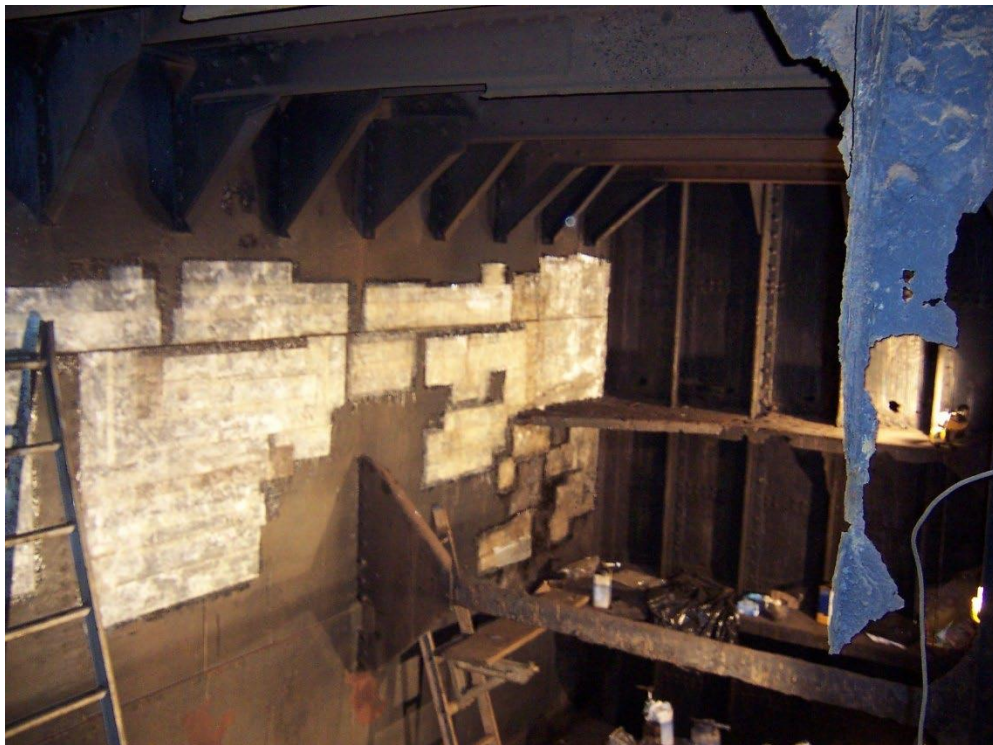
Wasted transverse bulkhead, indicative of conditions found throughout tank system. Bulkheads are Swiss cheese.
