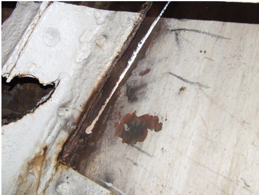
Wasted transverse frame/rivets and separated shell plating to starboard.
