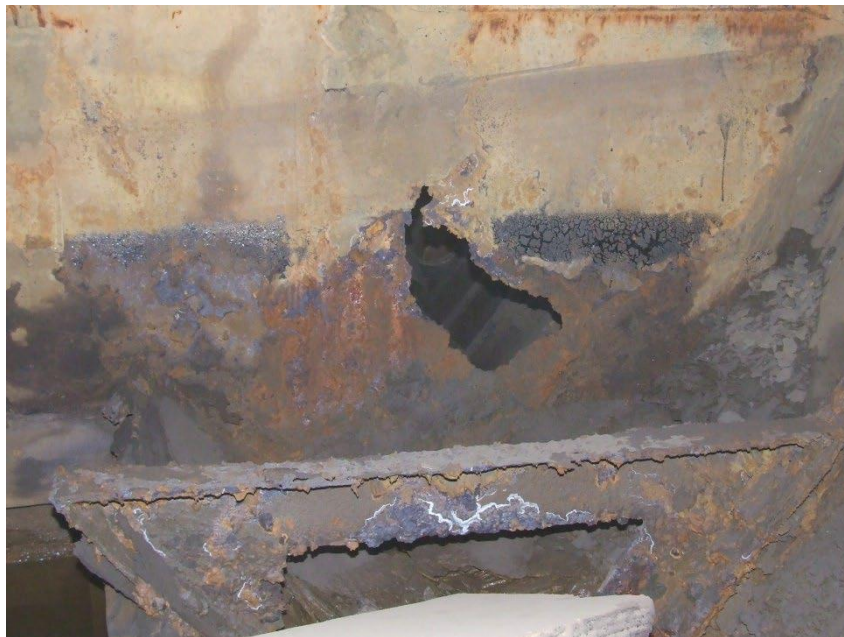
Holed main aft bulkhead into Tank #1 port.
