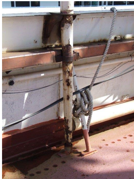
Wasted base of davit that previously supported the accommodation brow to port.
