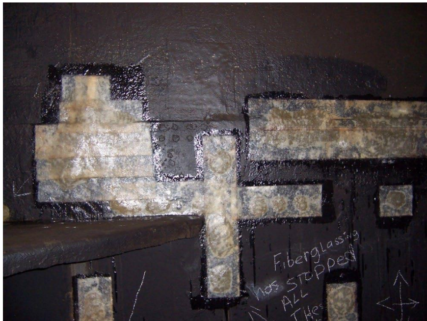
Patched bulkhead in Tank #3.
