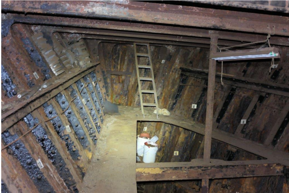
Intermediate level Aft Peak Tank.
