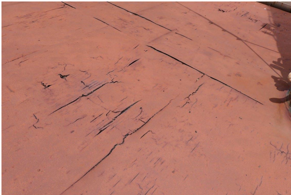
Plywood sheathed with fiberglass is over fir decking de-laminated with underlying plywood badly rotted throughout..
