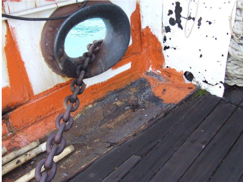
Concrete in waterways causing degradation to substrate. Notice wasted plating in right portion of photo.
