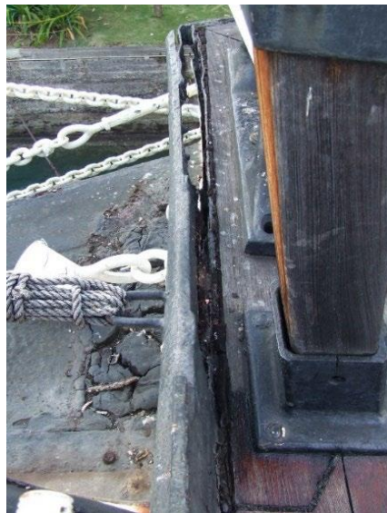
Leading edge of forecastle deck showing massive corrosion.
