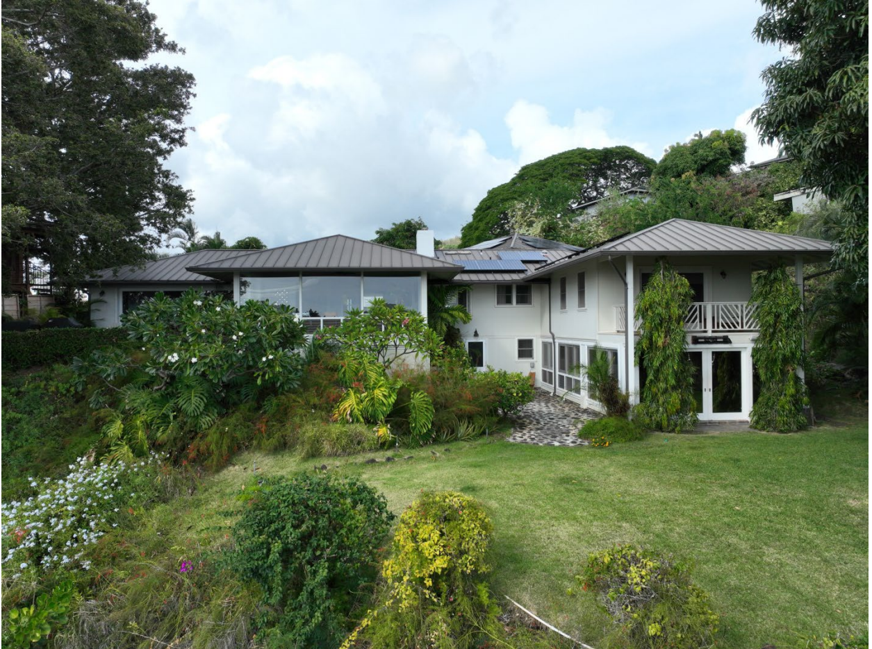
Drone view of the rear from the south
