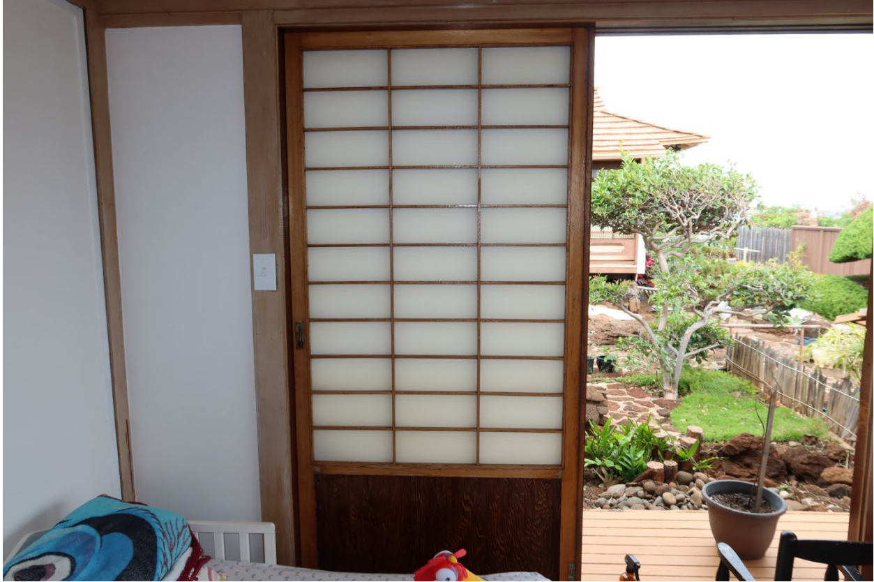
View of second floor north bedroom shoji from the east
