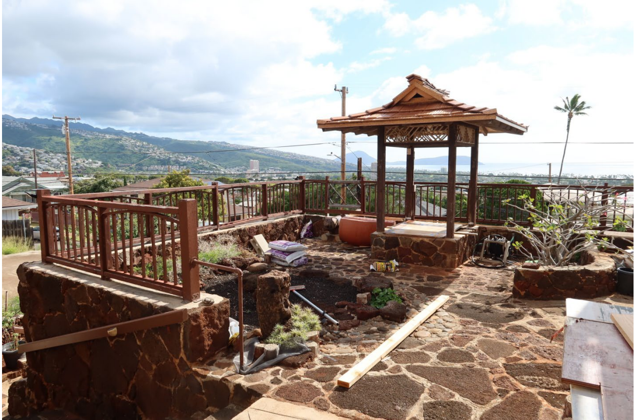
View of second terrace with dumb waiter terminus from the west
