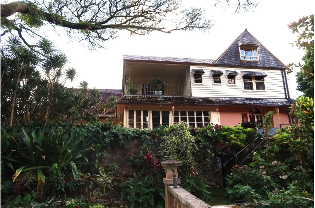
View of the rear of the house from the lower terrace from the east
