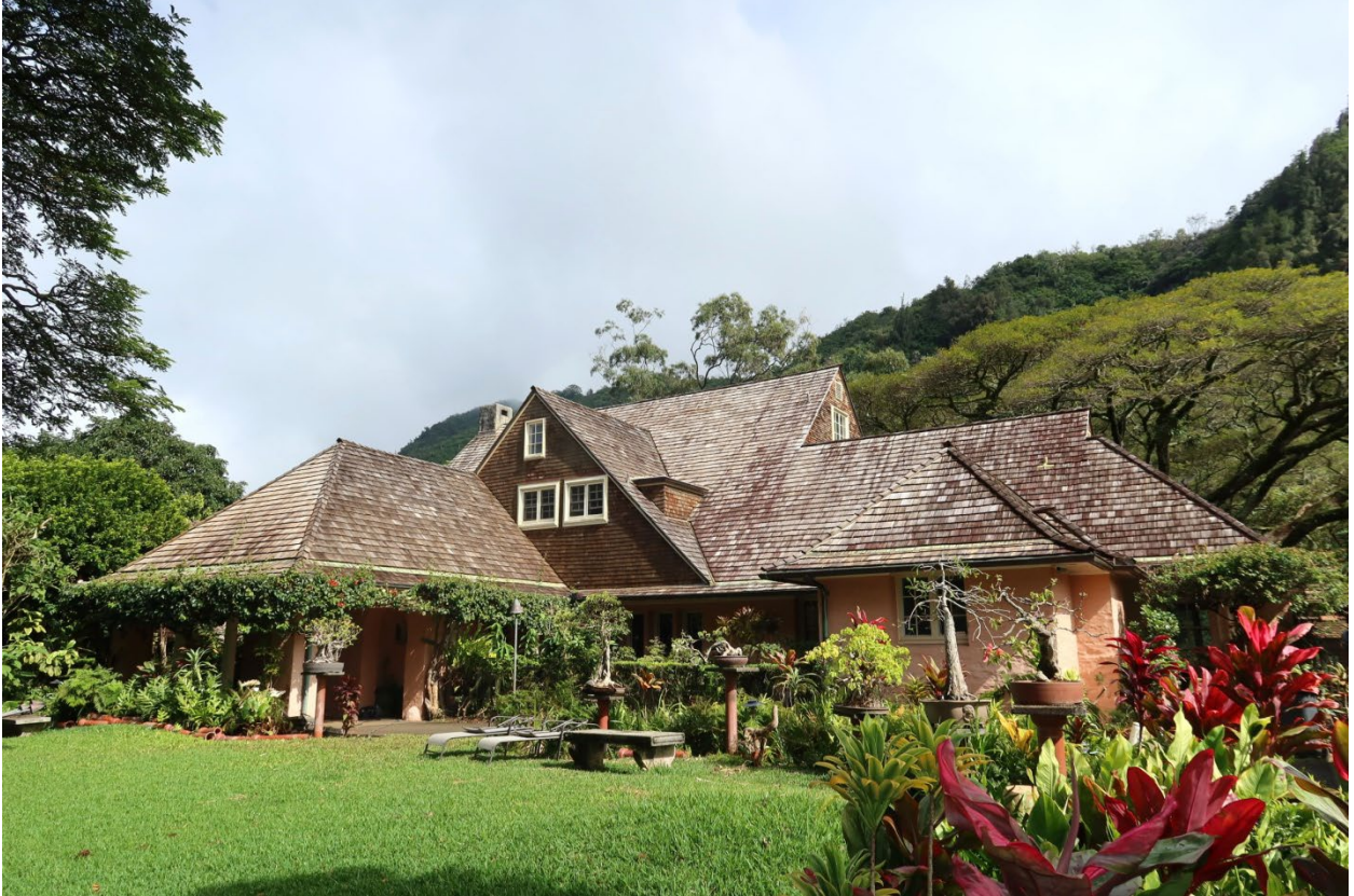
View of the front from the southwest
