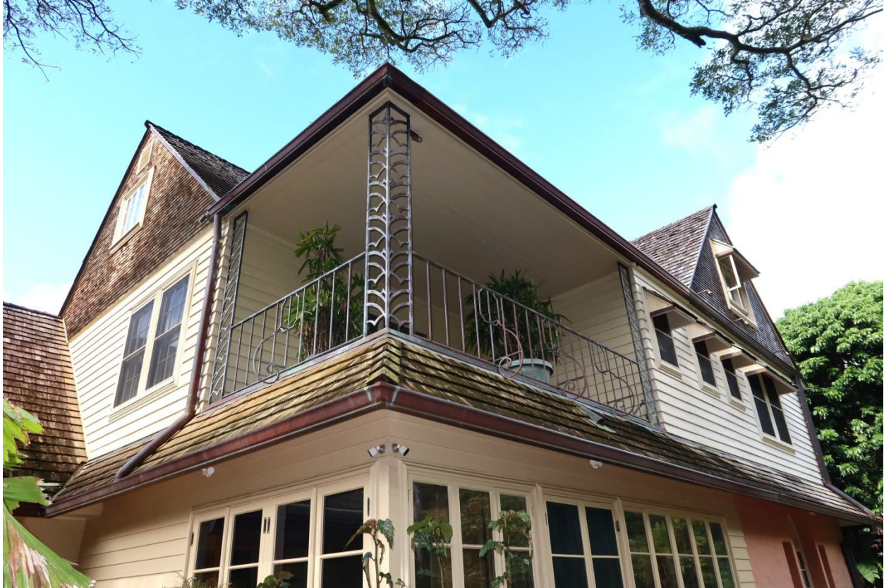
View of master bedroom balcony from the southeast
