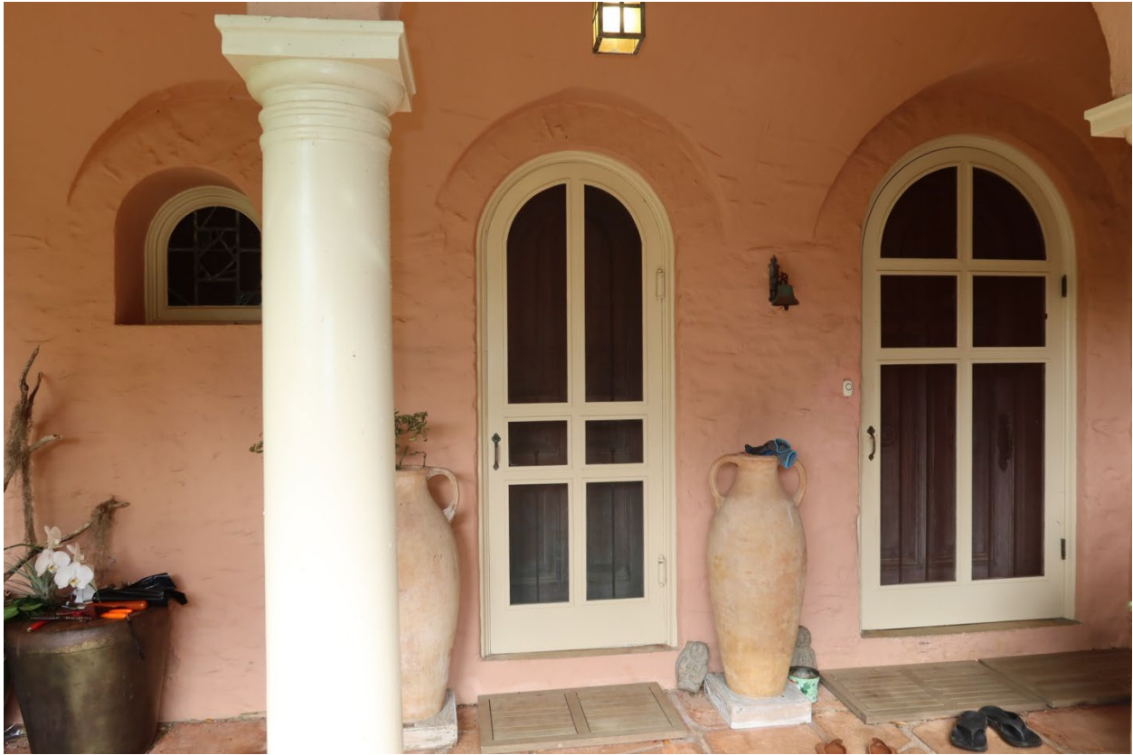
View the doors to foyer and study from the south
