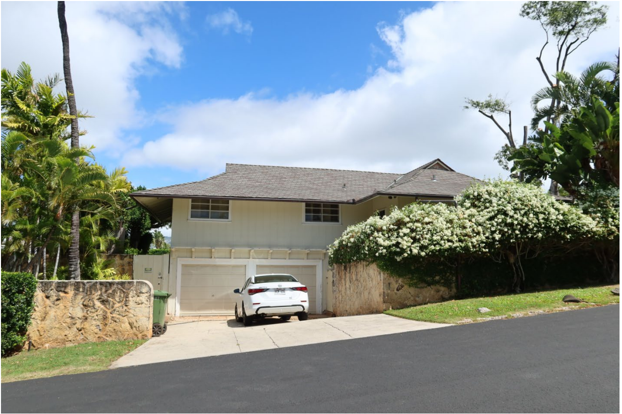
View of the side of the house from the south
