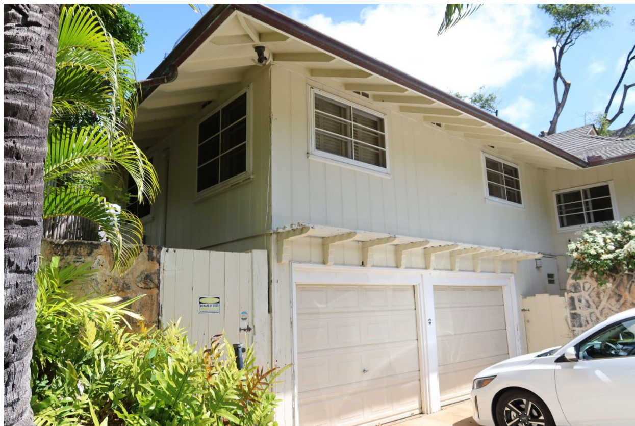
View of the garage and south bedroom wing from the southwest
